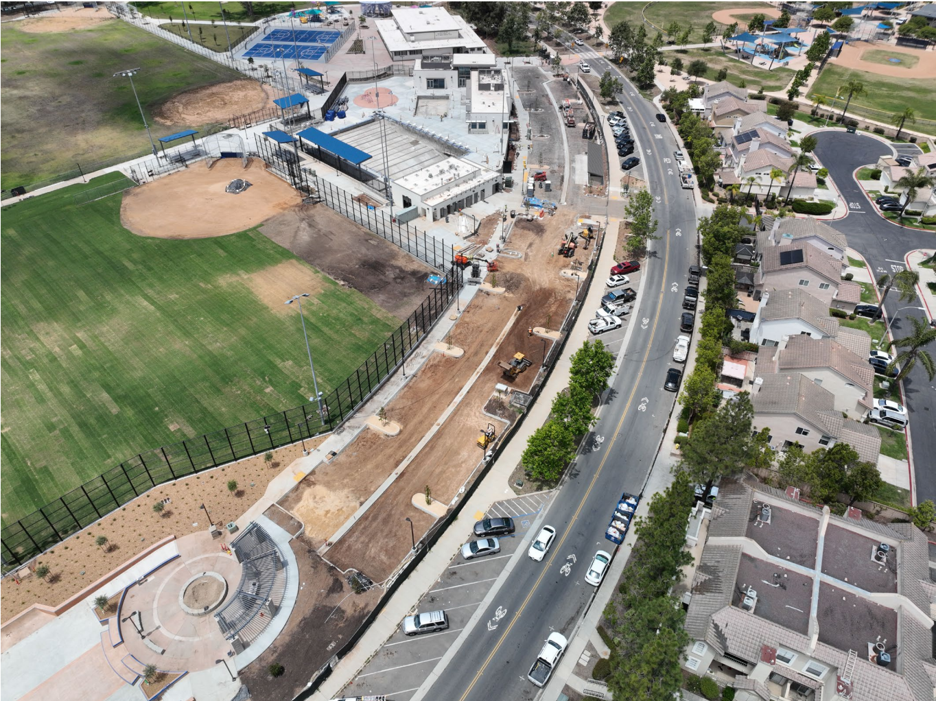
Ongoing concrete placement for new parking lot ribbon gutter.
