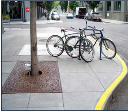
Curb bulb-outs reduce the crossing distance for pedestrians and provided space for amenities such as bicycle parking, landscaping and street furniture.
