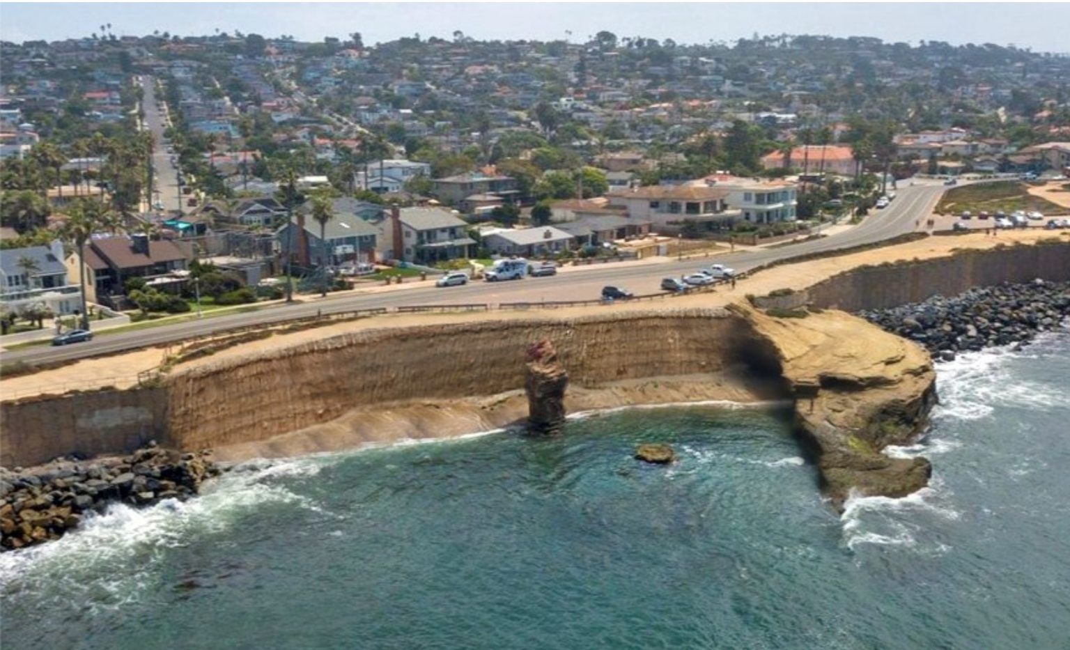
Rendering of a Shotcrete Tieback Wall
