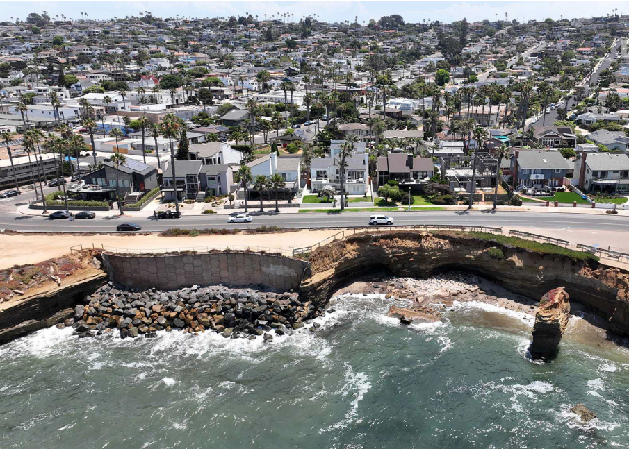
Example: Existing Engineered Seawall
