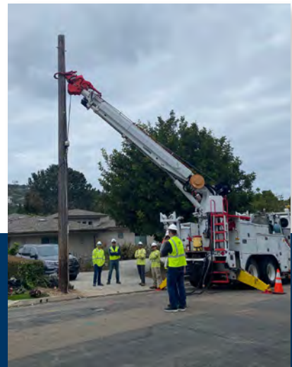
Once all cables and wires have been cleared and only poles remain, overhead poles are removed.
