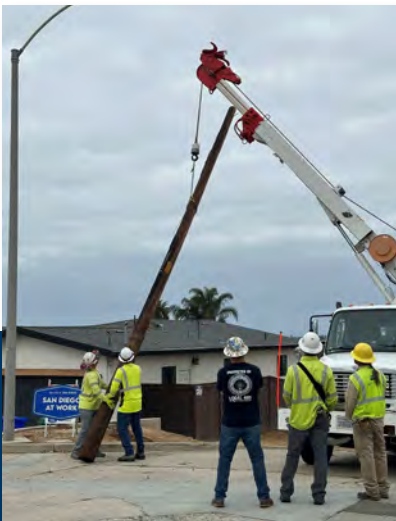
Once all cables and wires have been cleared and only poles remain, overhead poles are removed.
