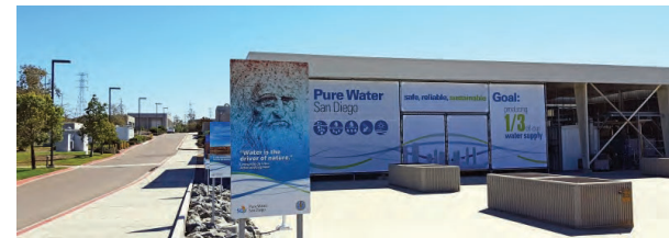
Pure Water San Diego Demonstration Facility 2017
