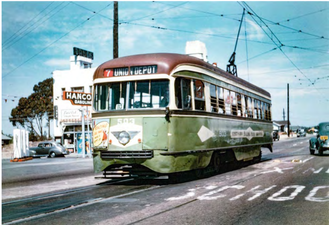
Figure 51. A streetcar on Line 7 at the intersection of University and Euclid avenues in 1947. Source: Bob McKay, www.railwaypreservation.com .
