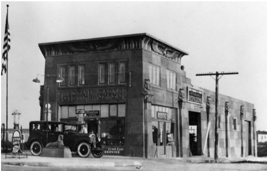
Figure 58: Egyptian Garage (4749 University Avenue), built 1923-25. Source: Los Angeles Public Library Legacy Collection.
