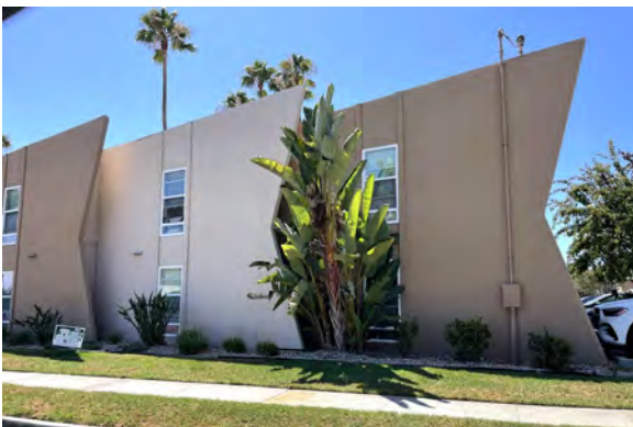
Figure 106: Mid-Century Modern apartment building (6271 Madeline Street, built 1963) with a unique staggered façade profile.
