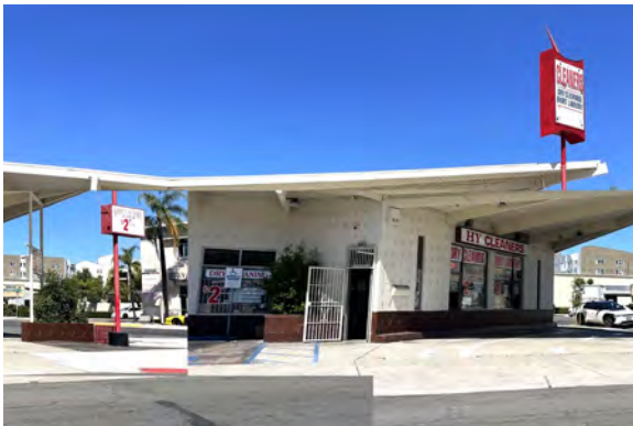
Figure 81: 4441 El Cajon Boulevard (c.1953-64), Mid-Century Modern commercial building with a drive-thru under a triangular canopy.
