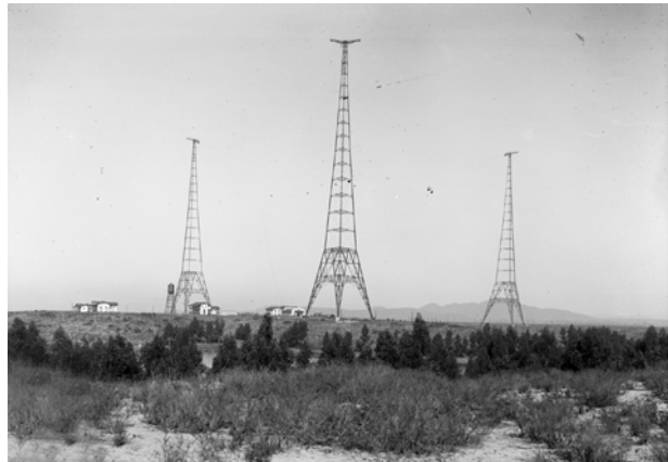
Figure 117: The three towers of the Chollas Heights Naval Radio Station, with some service buildings in background, ca. 1916. Source: UG 21-11.04, Chollas Heights Naval Radio Station Collection, Archives Branch, Naval History and Heritage Command, Washington, DC.
