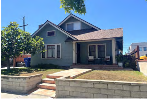
Figure 14: The Wahrenbrock Residence at 4752 Felton Street (1912) in Normal Heights.
