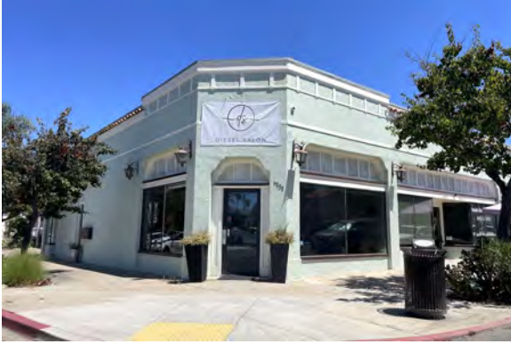
Figure 62: Neighborhood commercial building at 4222 Adams Avenue (ca. 1930).
