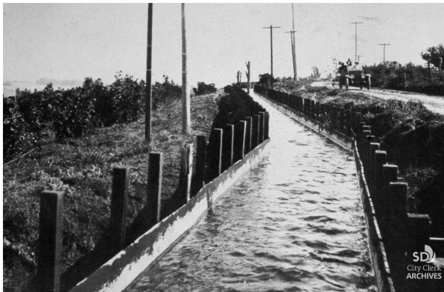
Figure 4: An example of the open flume at an unknown location in 1905 as built by the San Diego Flume Company. Since demolished. Source: San Diego City Clerk Archives.
