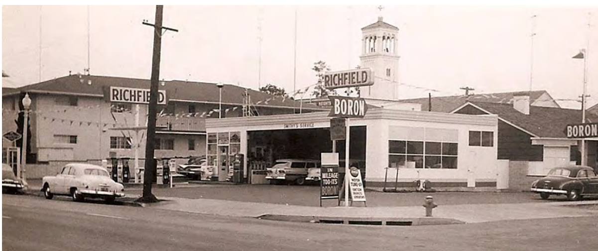
Figure 74: Smitty's Service, serving Richfield gas, at 3441 Adams Avenue, c. 1940s. Source: Smitty's Service, smittyservice.net.
