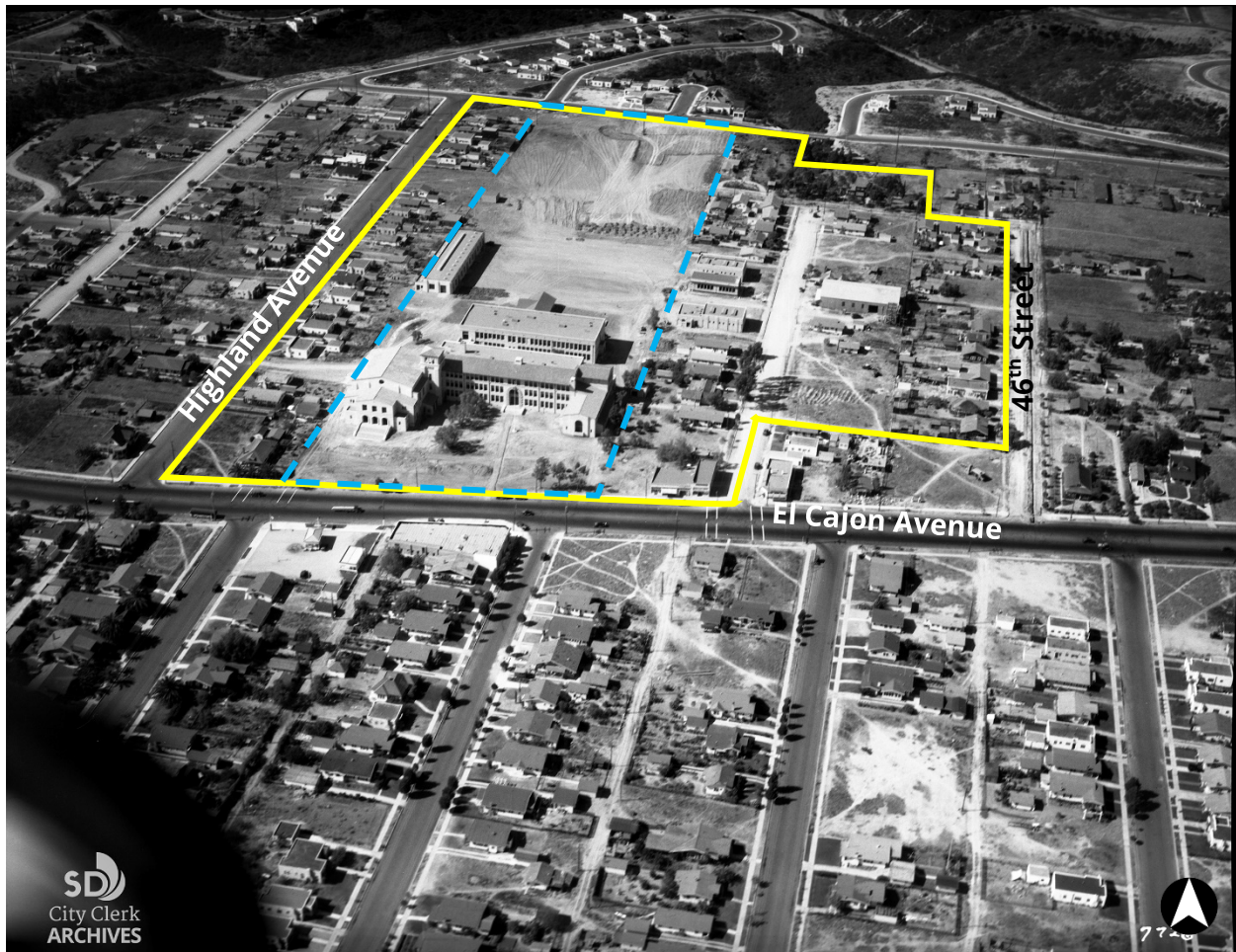
Figure 113: Herbert Hoover High School (4474 El Cajon Boulevard) in the Kensington-Talmadge area in 1930. Initial campus boundary shown in dashed blue line; campus has been expanded to the present day to include land within yellow outline. None of the original buildings are extant. Source: San Diego City Clerk Archives. Edited by Page & Tunbull.
