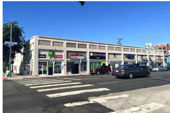
Figure 26: Former East San Diego City Hall, which has been substantially altered through various alterations (removal of parapet and ornamental detailing infilling open bays, redesign of storefronts) to the point of a loss of historic integrity.
