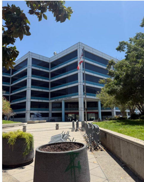
The presence of the Police Department headquarters (above) and Fire Department station benefit public safety efforts, but additional police and fire stations will be needed to maintain service levels in future years.
