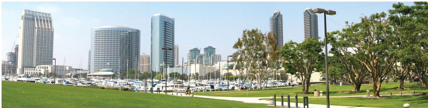
Embarcadero Marina Park South — one of the largest parks downtown, but difficult to access on foot.
