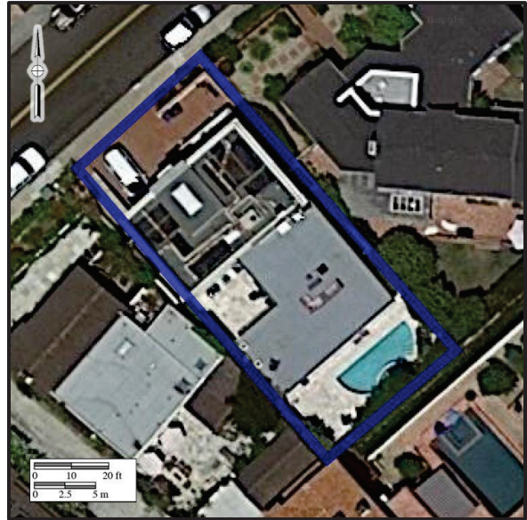
Plate 2.0–1: Aerial view of the current development at 1855 Spindrift Drive.
