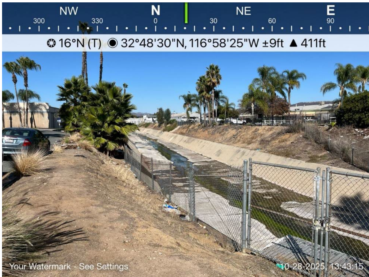
Photo 6. Work Location 382+78 and a view of NWW-ALT-02; facing north. October 28, 2025.
