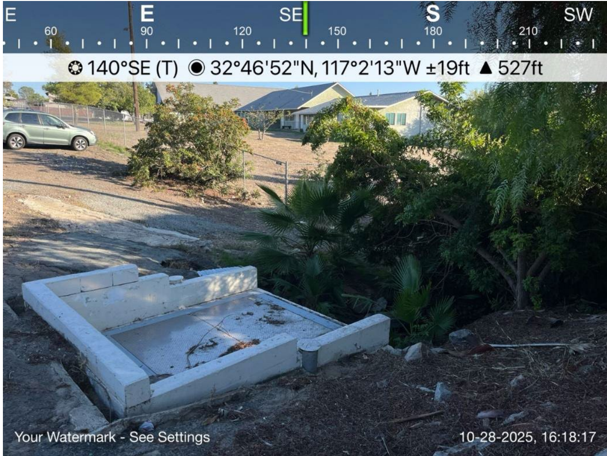
Photo 16. Work Location 644+21 and view of NWW-ALT-08; facing southeast. October 28, 2025.
