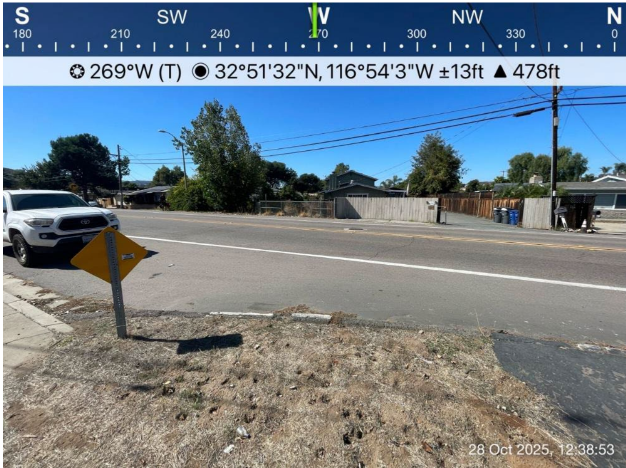
Photo 9. Work Location 40+29, with NWW-ALT-03 behind the photographer. View facing west. October 28, 2025.
