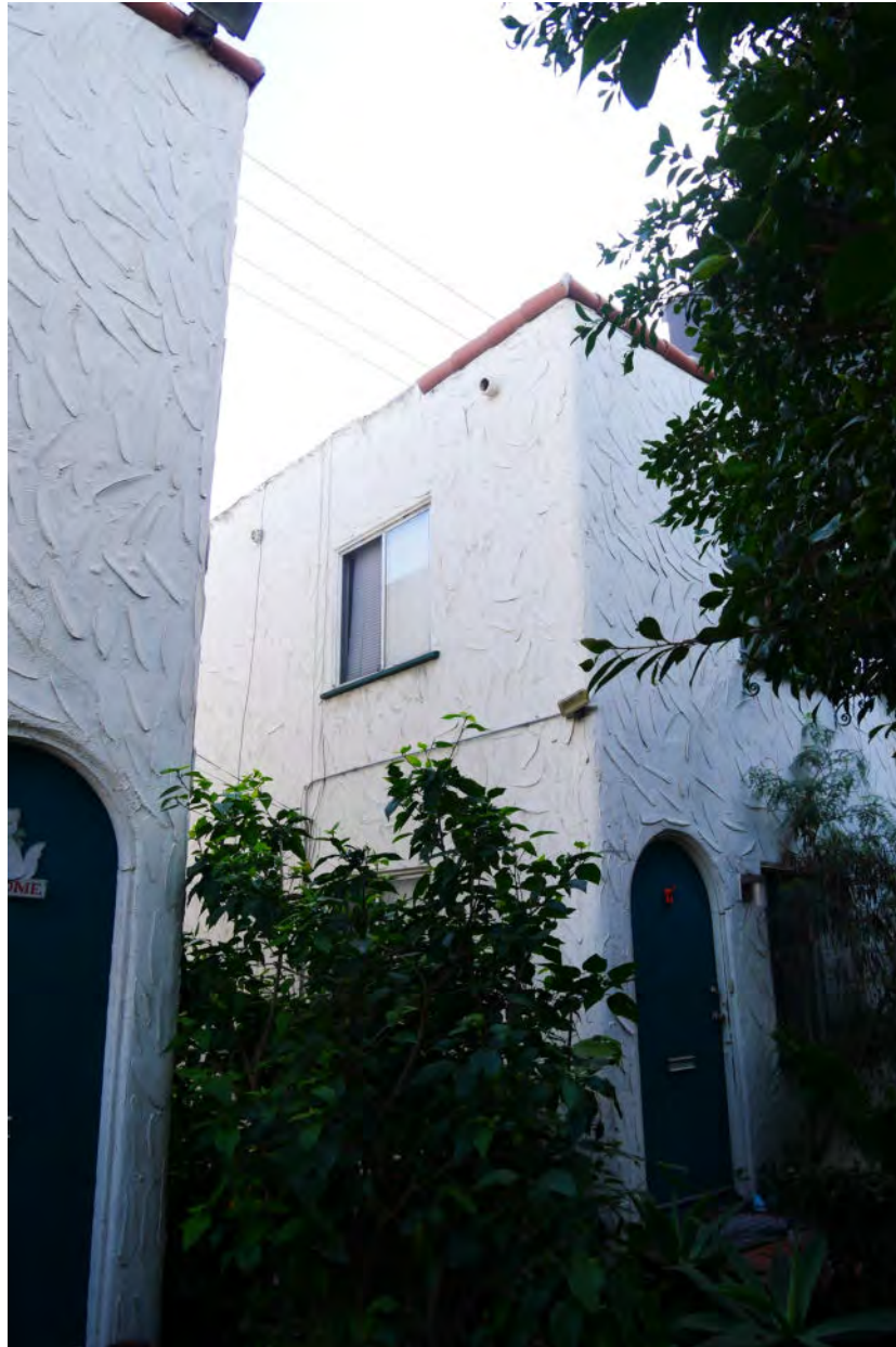
Photograph #41: north elevation of two-story duplex
