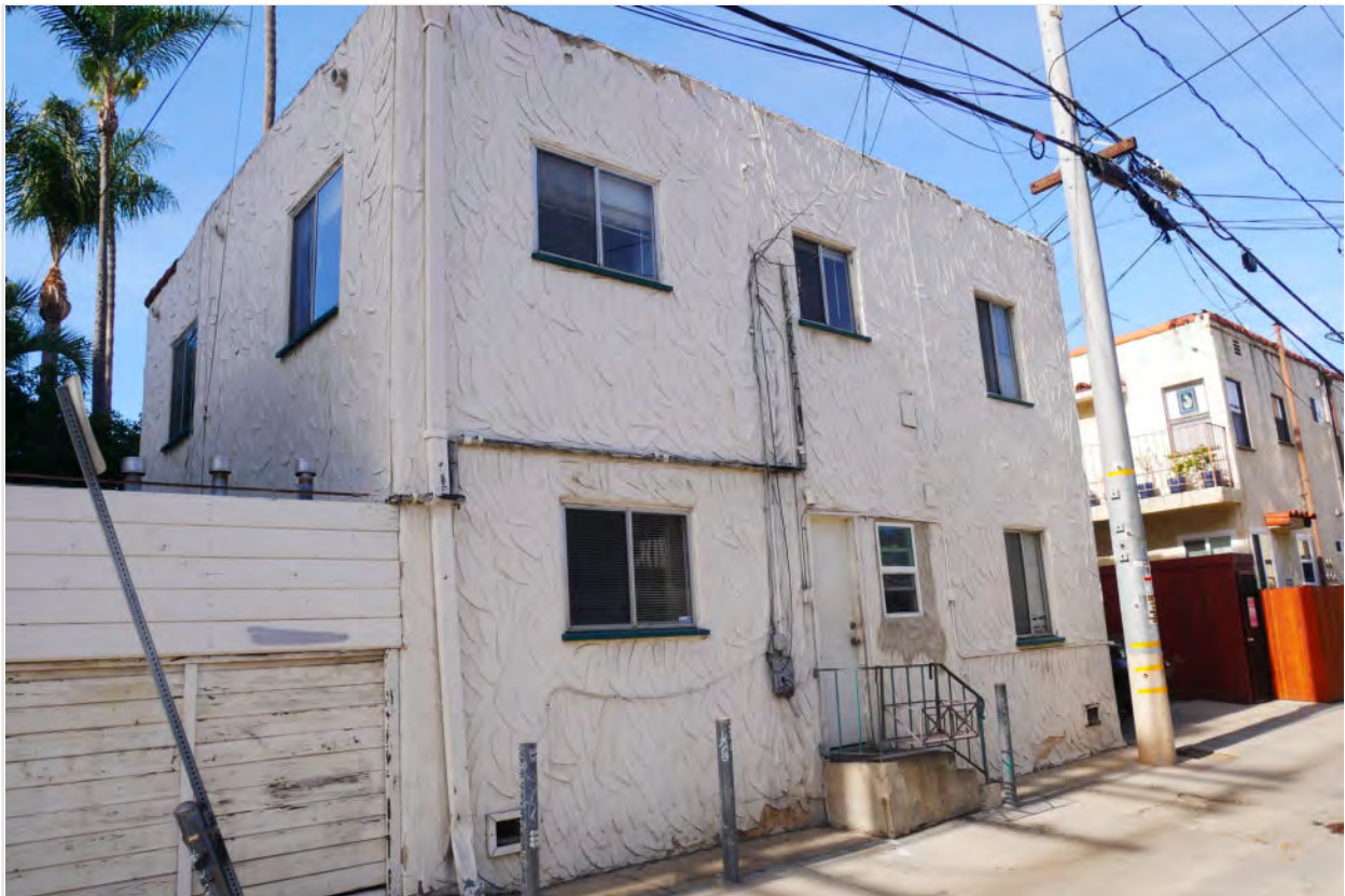
Photograph #31: East elevation at alley
