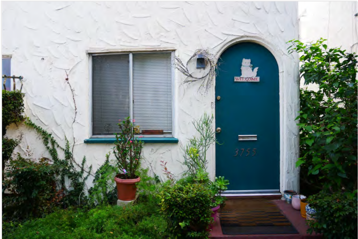
Photograph #39: South elevation. One-story duplex, 3755 Fourth Elevation
