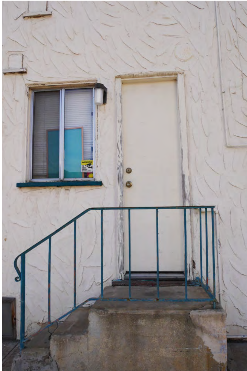
Photograph #32: East elevation, rear building
