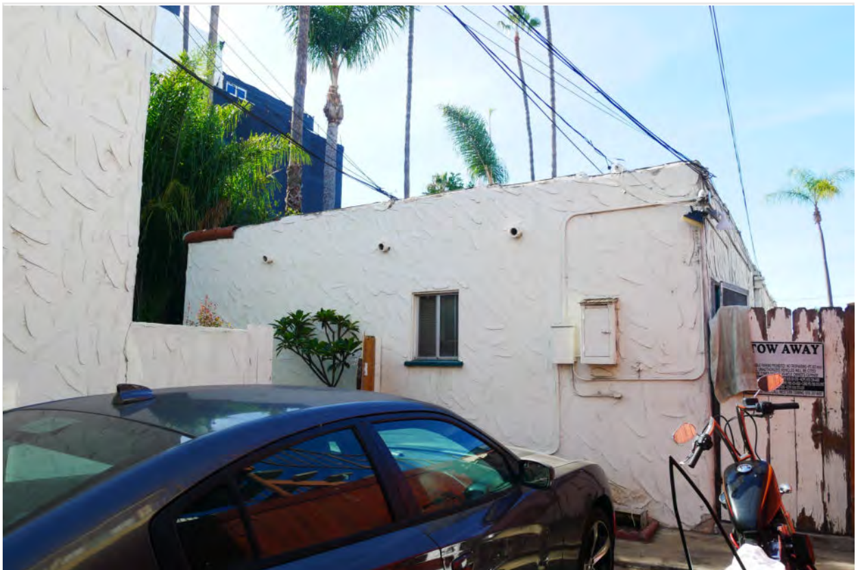
Photograph #34: East elevation of one-story building
