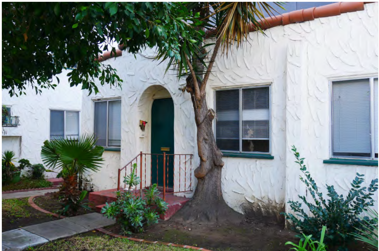
Photograph #12: North elevation duplexes
