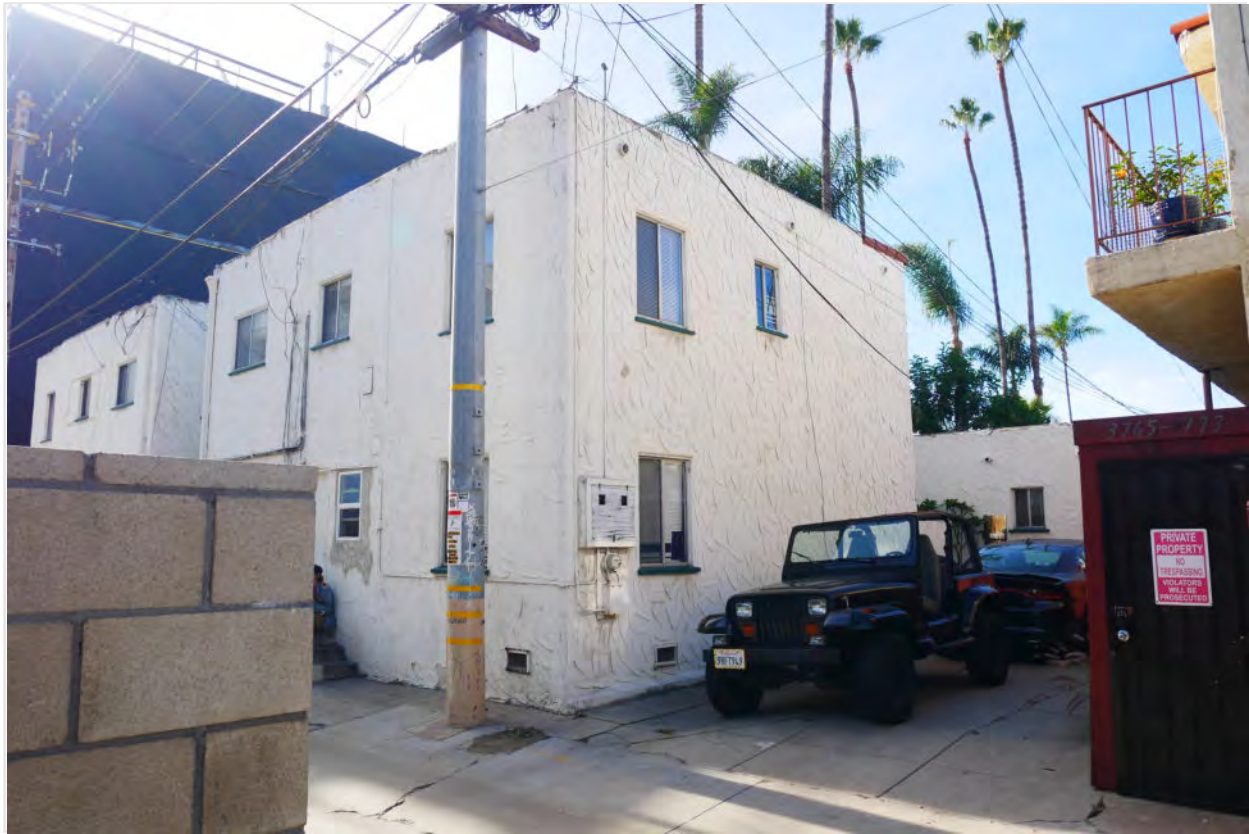
Photograph #33: Northeast corner of site
