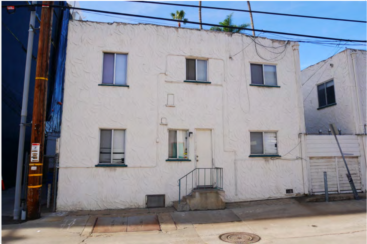
Photograph #30: East elevation at alley
