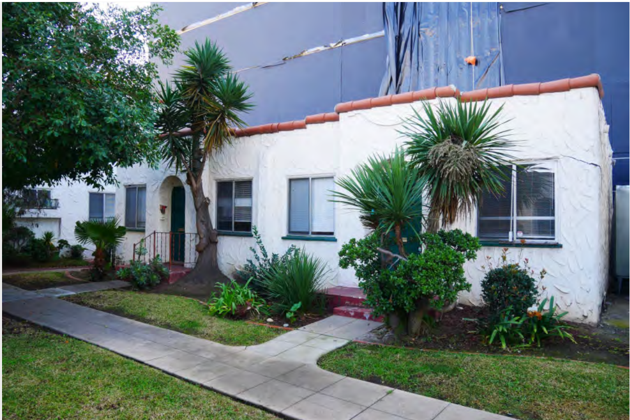
Photograph #10: North elevation duplexes
