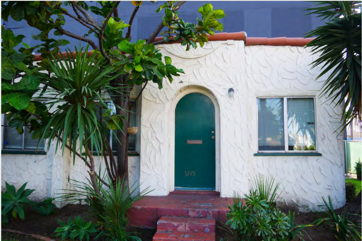
Photograph #9: North elevation duplexes
