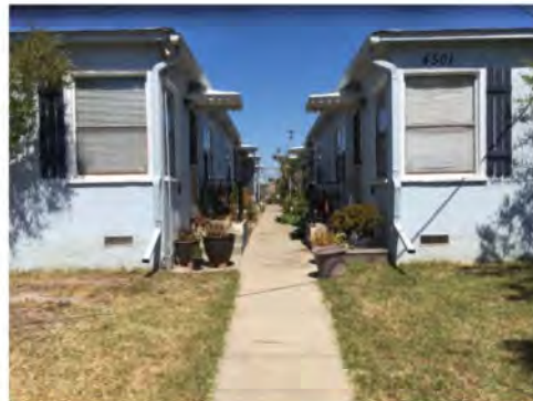
Full bungalow court at 4501 Illinois Street with open plan, narrow court, attached units.
