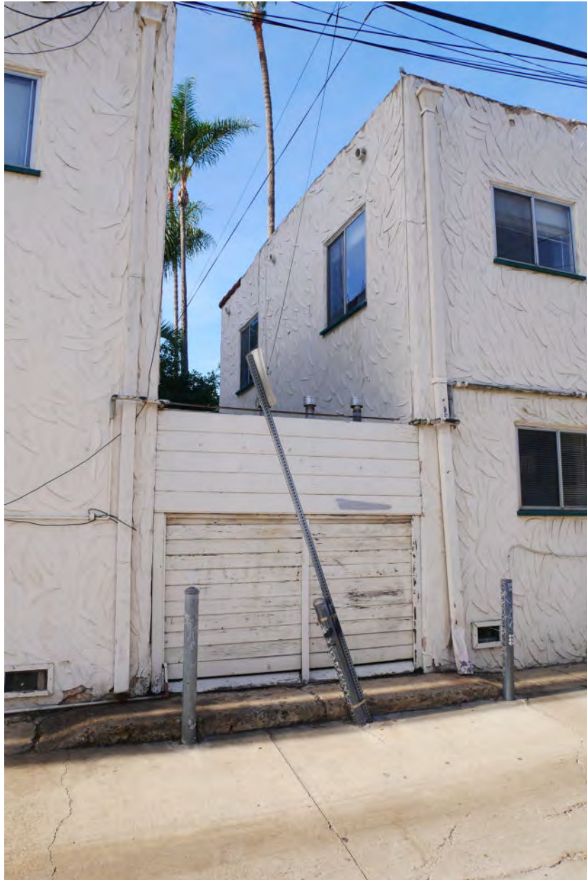
Photograph #29: East elevation at alley
