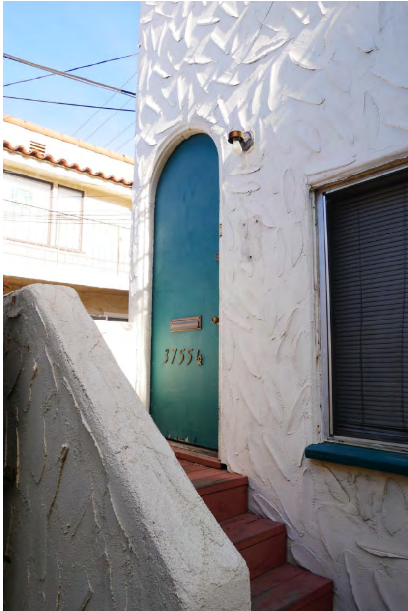
Photograph #36: South elevation two-story duplex entry
