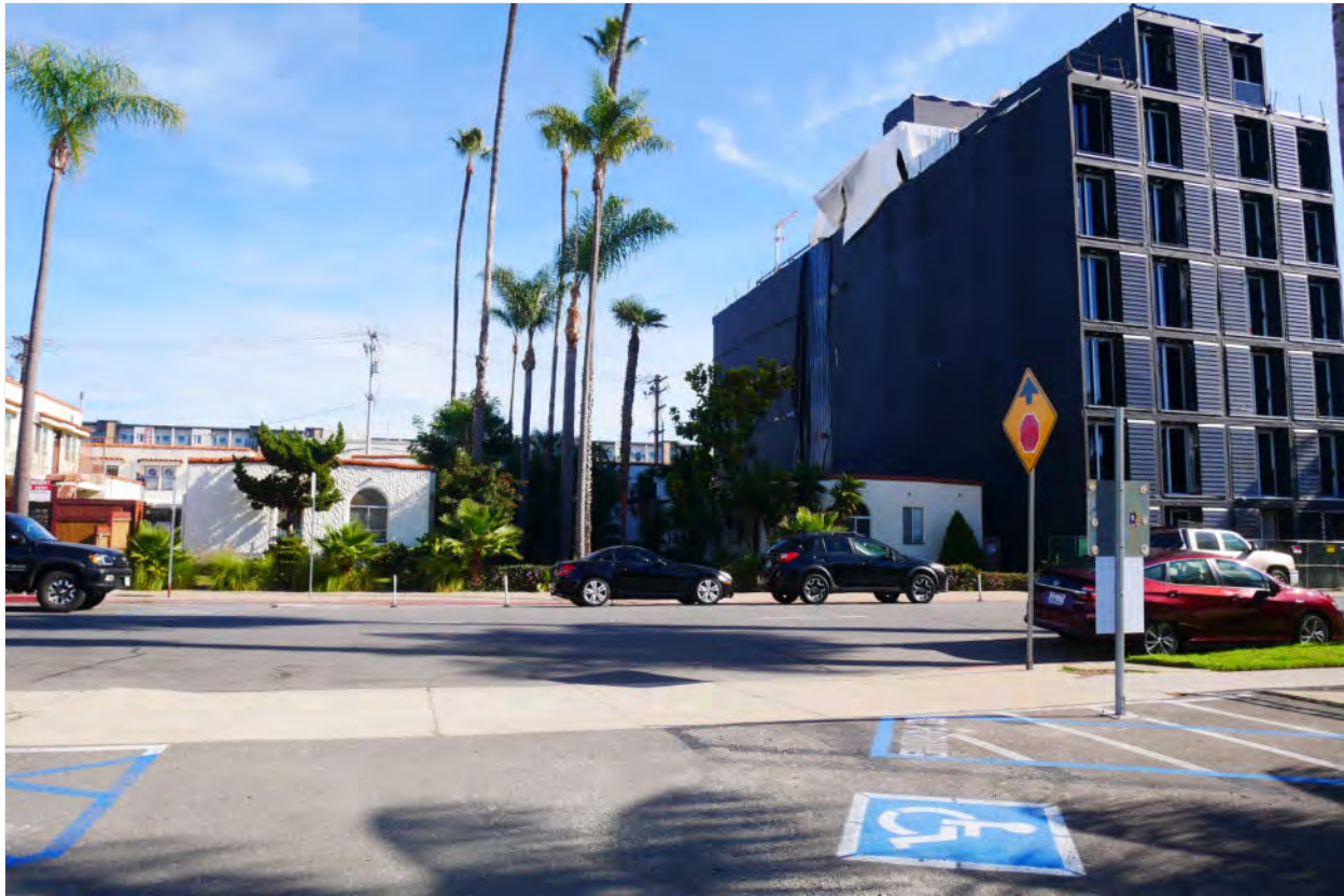
Photograph #1: West elevation, facing Fourth Avenue
