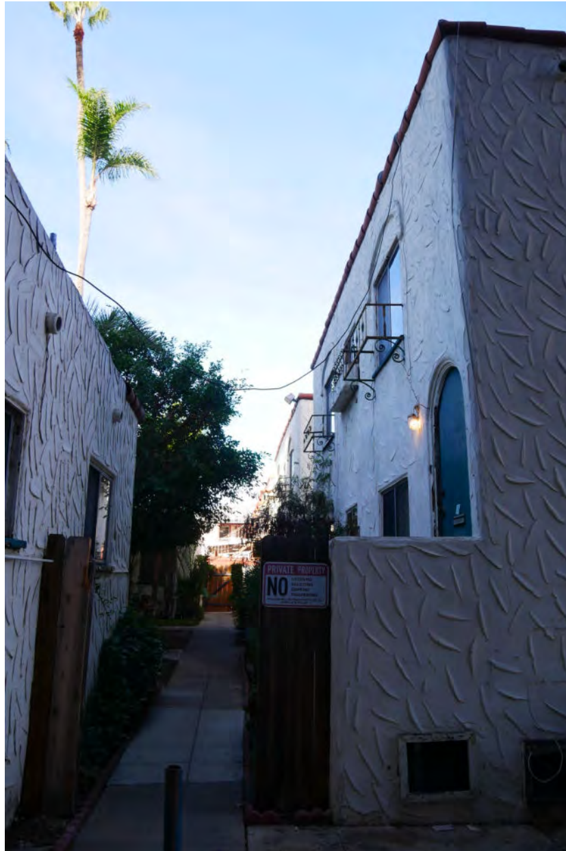
Photograph #48: Space between one-story and two-story buildings
