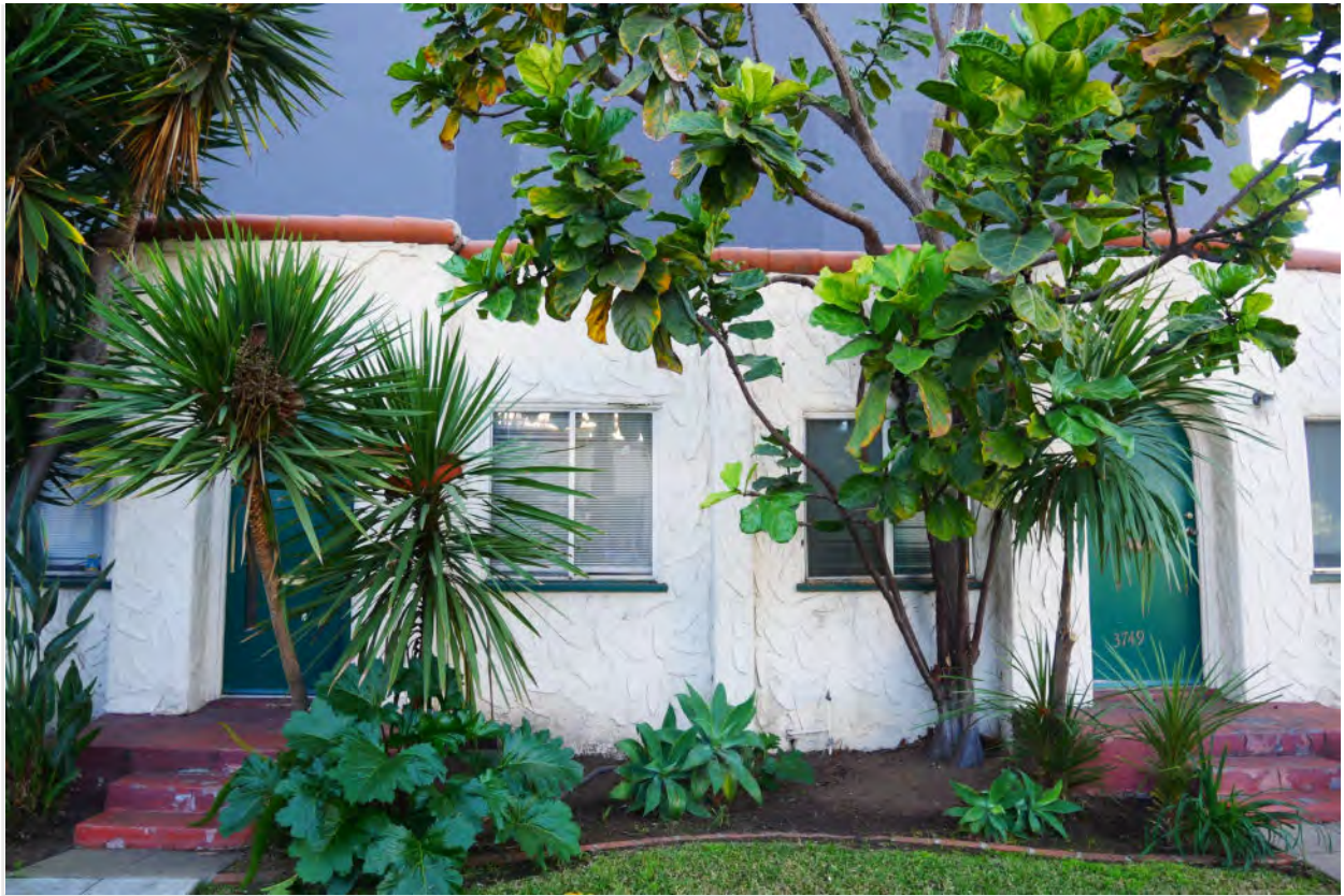
Photograph #11: North elevation duplexes
