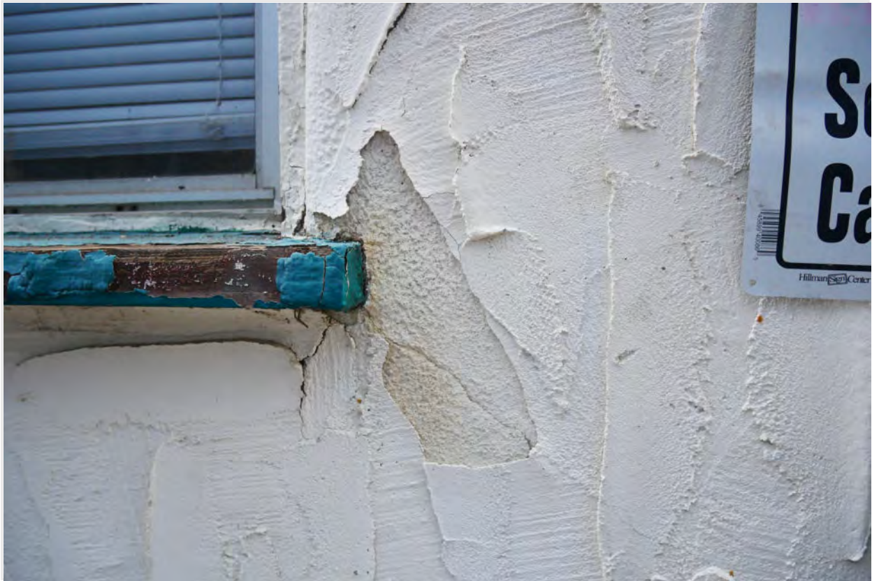
Photograph #49: Non-original heavy textured stucco failing and exposed original stucco texture visible
