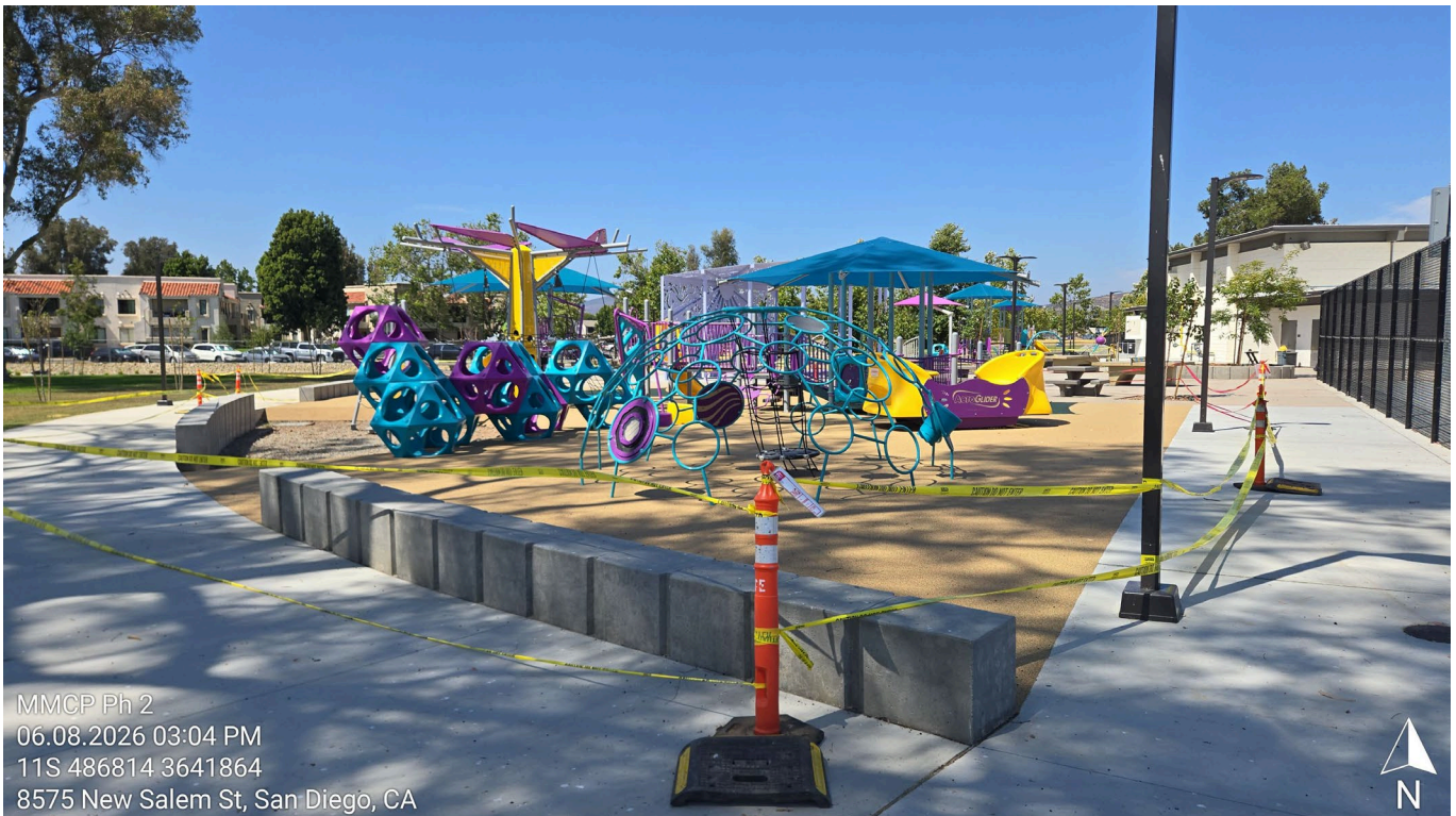
Installation of the rubberized safety surfacing in the children's play areas.
