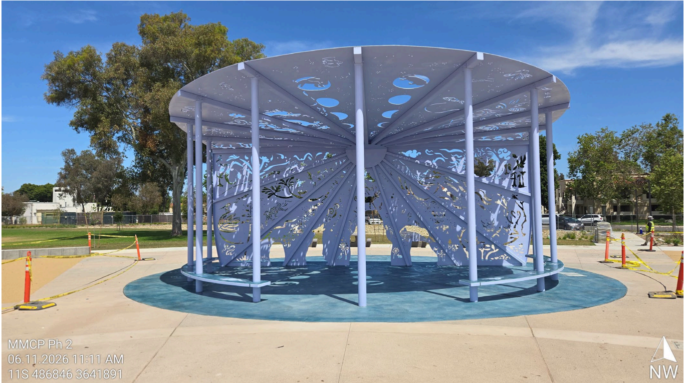
Blue concrete staining for the public art base.
