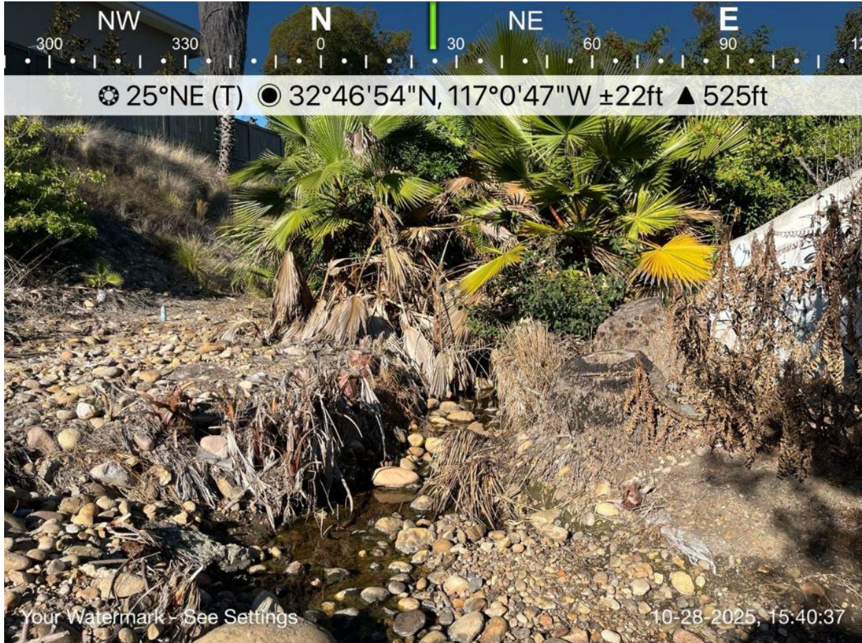
Photo 12. Work Location 555+79 is to the left of the photo of NWW-ALT-06, a channel associated with a culvert under Fletcher Parkway. View facing north. October 28, 2025.
