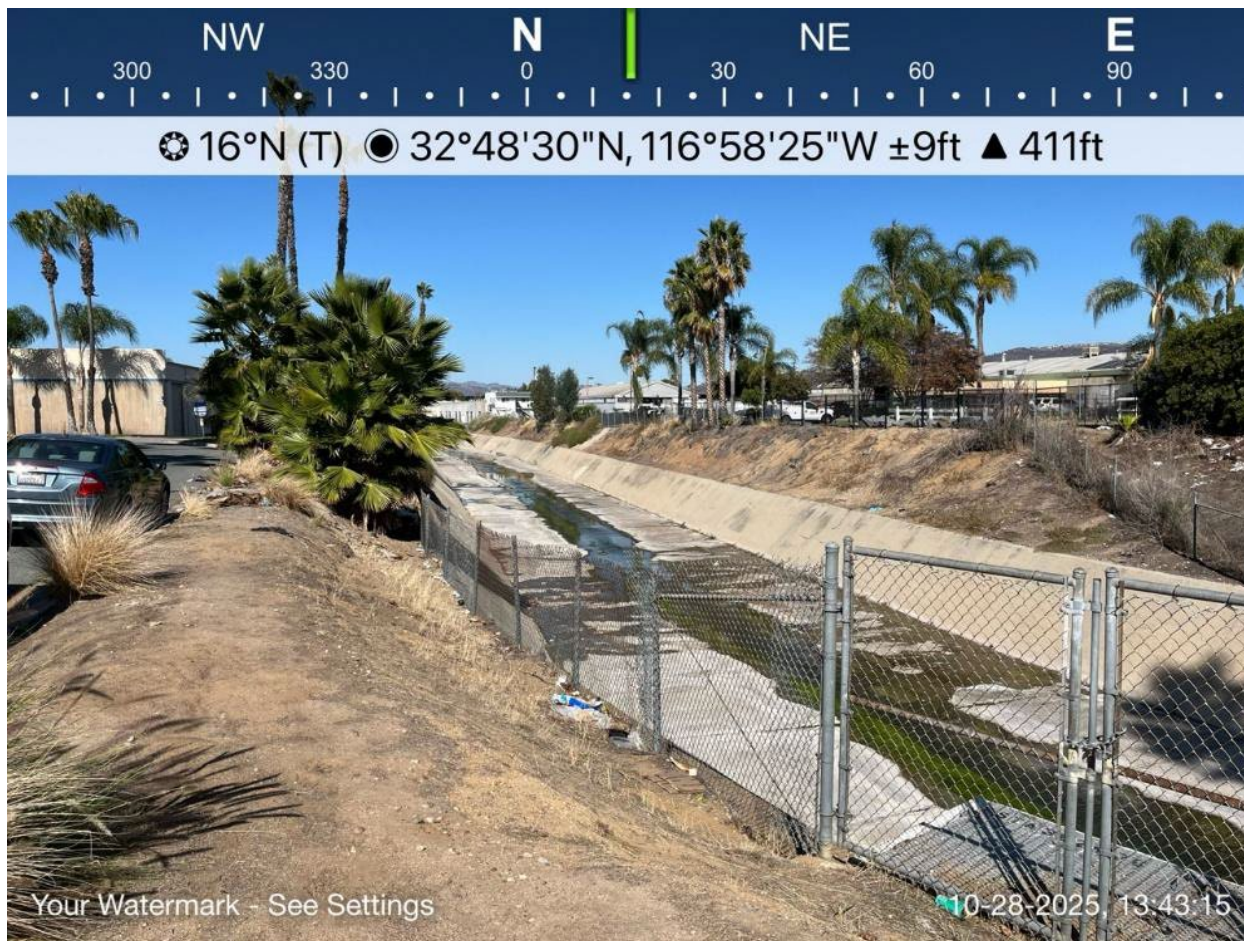
Photo 4. Work Location 382+78 and a view of NWW-ALT-02; facing north. October 28, 2025.
