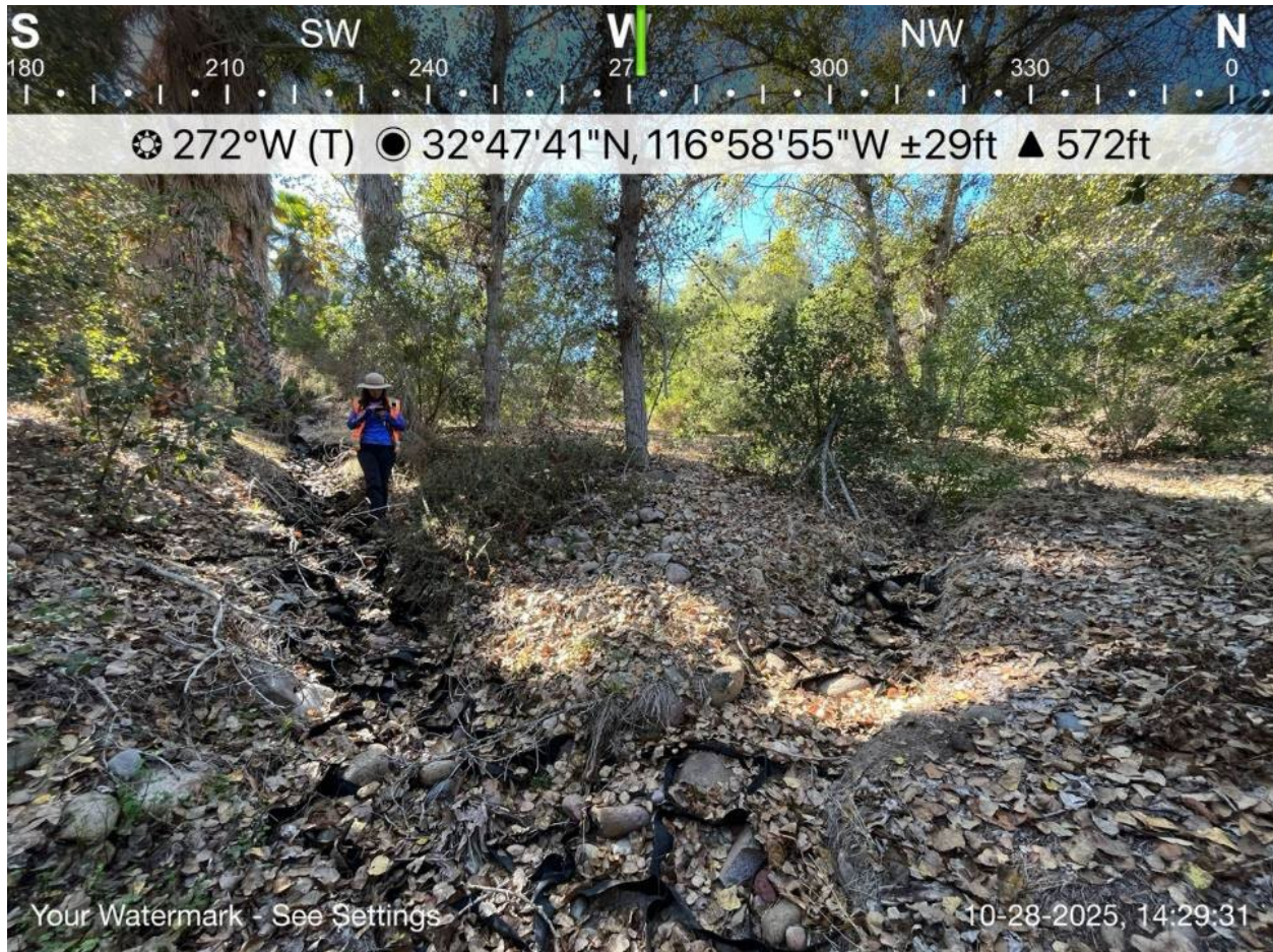
Photo 9. Work Location 439+20. Convergence of intermittent channel NWW-ALT-04 and ephemeral channel NWW-ALT-05; both provide surface flow connections to stormwater culverts. Note existing geogrid and rock installed to reduce erosion. View facing west. October 28, 2025.
