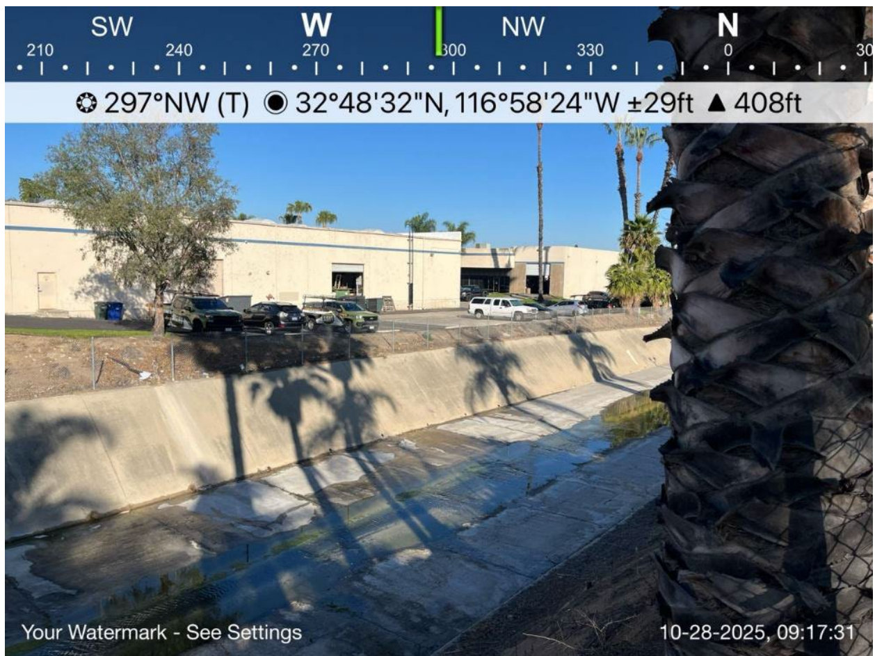
Photo 2. Work Location 380+15 and a view of NWW-ALT-02, a channelized waterway; facing west. October 28, 2025.
