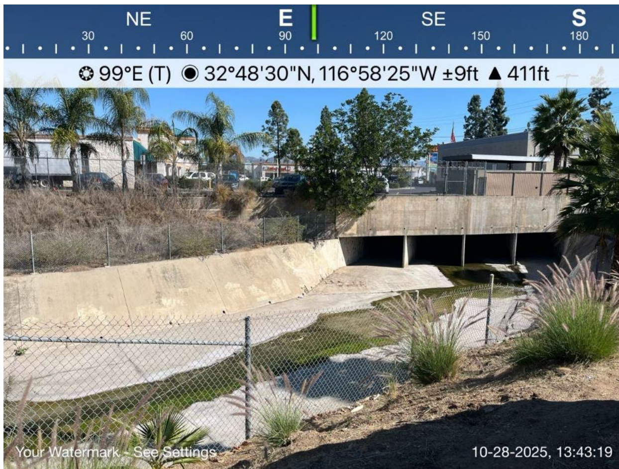
Photo 5. Work Location 382+78 and a view of NWW-ALT-02; facing east. October 28, 2025.
