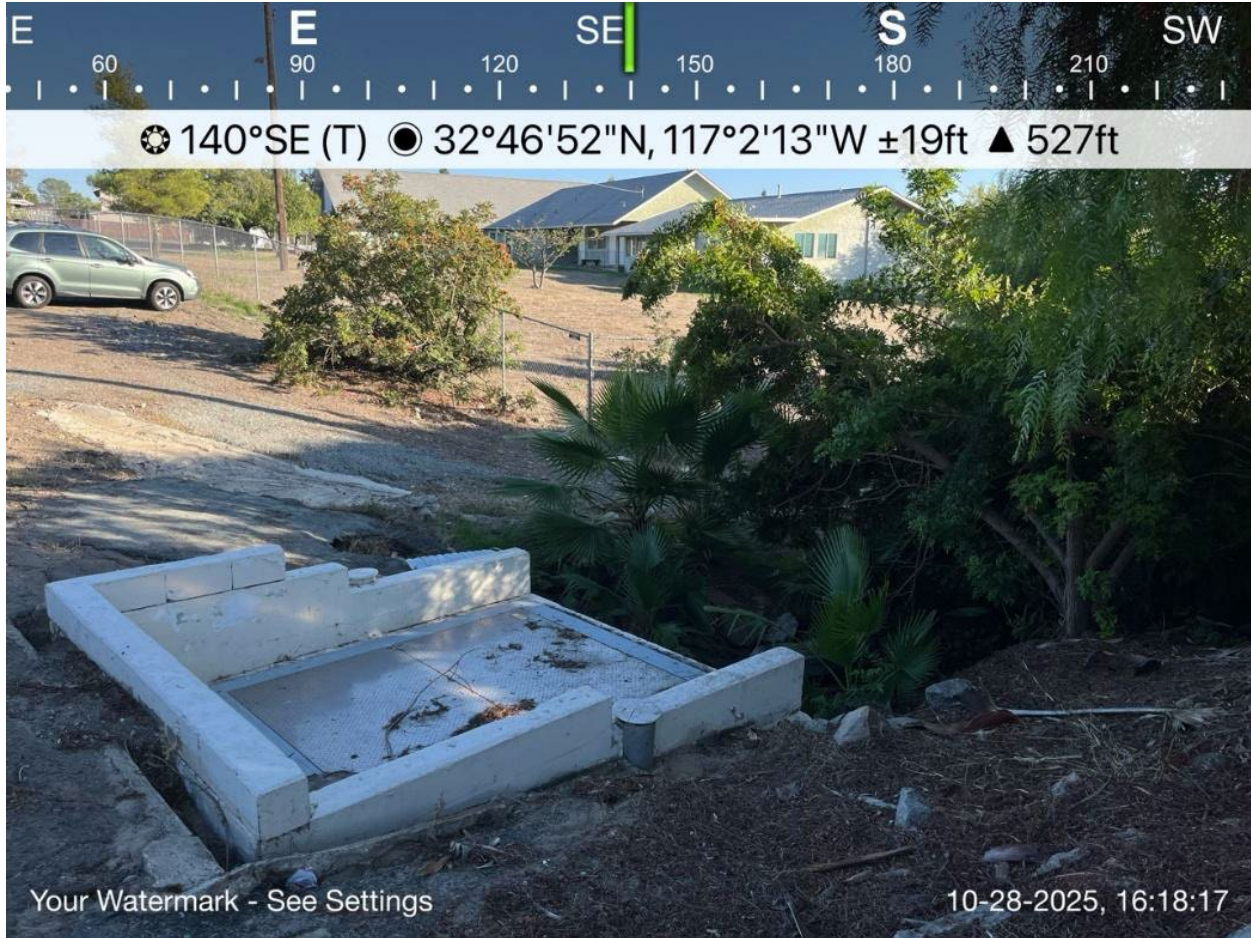
Photo 14. Work Location 644+21 and view of NWW-ALT-08; facing southeast. October 28, 2025.
