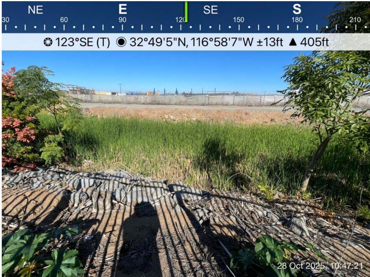
Photo 1. Work Location 345+20 and a view of NWW-ALT-01, a canal constructed between W Bradley Avenue and Floyd Smith Drive; facing southeast. October 28, 2025.
