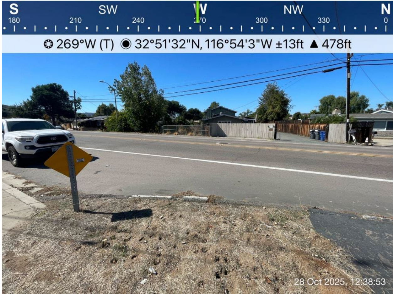
Photo 7. Work Location 40+29, with NWW-ALT-03 behind the photographer. View facing west. October 28, 2025.
