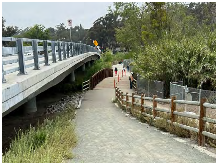
Photo 20: Looking north on the east side of the Willow Street Bridge toward where Feature 1a enters the main Sweetwater River Channel (Feature 1) on left of trail and pedestrian bridge (May 26, 2022).
