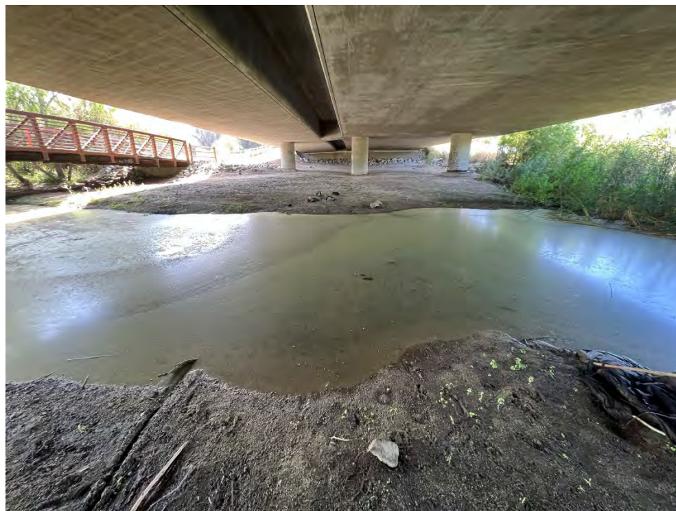
Photo 6: Looking south across the Sweetwater River to the south abutment of the Willow Street Bridge (July 20, 2022).
