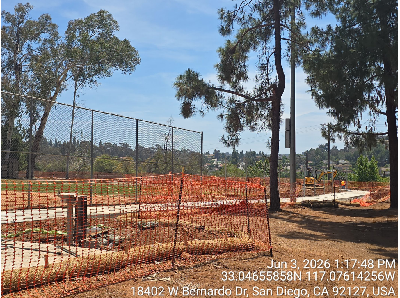
Concrete placement behind Field 8.
