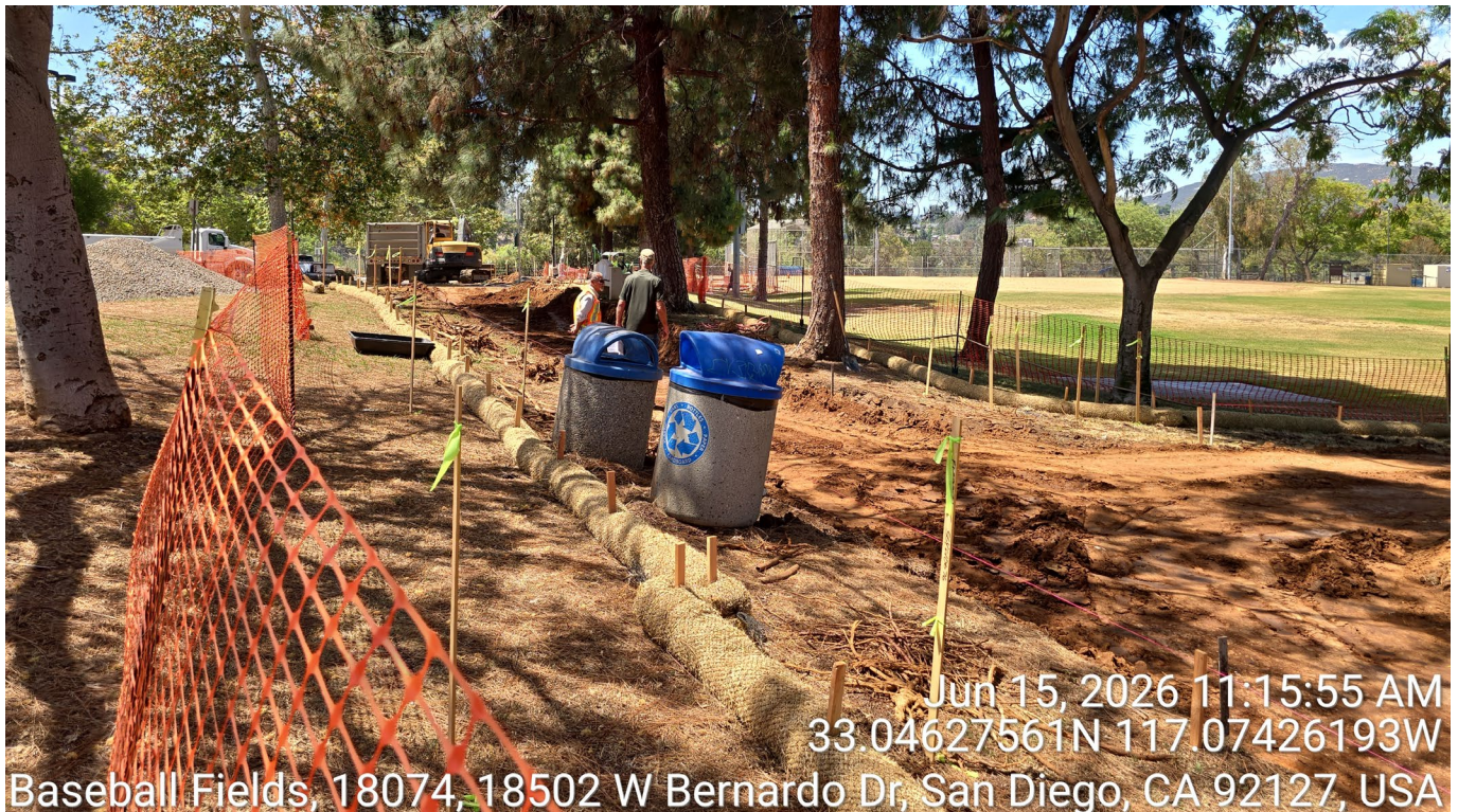
Grading at the north-east of Field 7.
