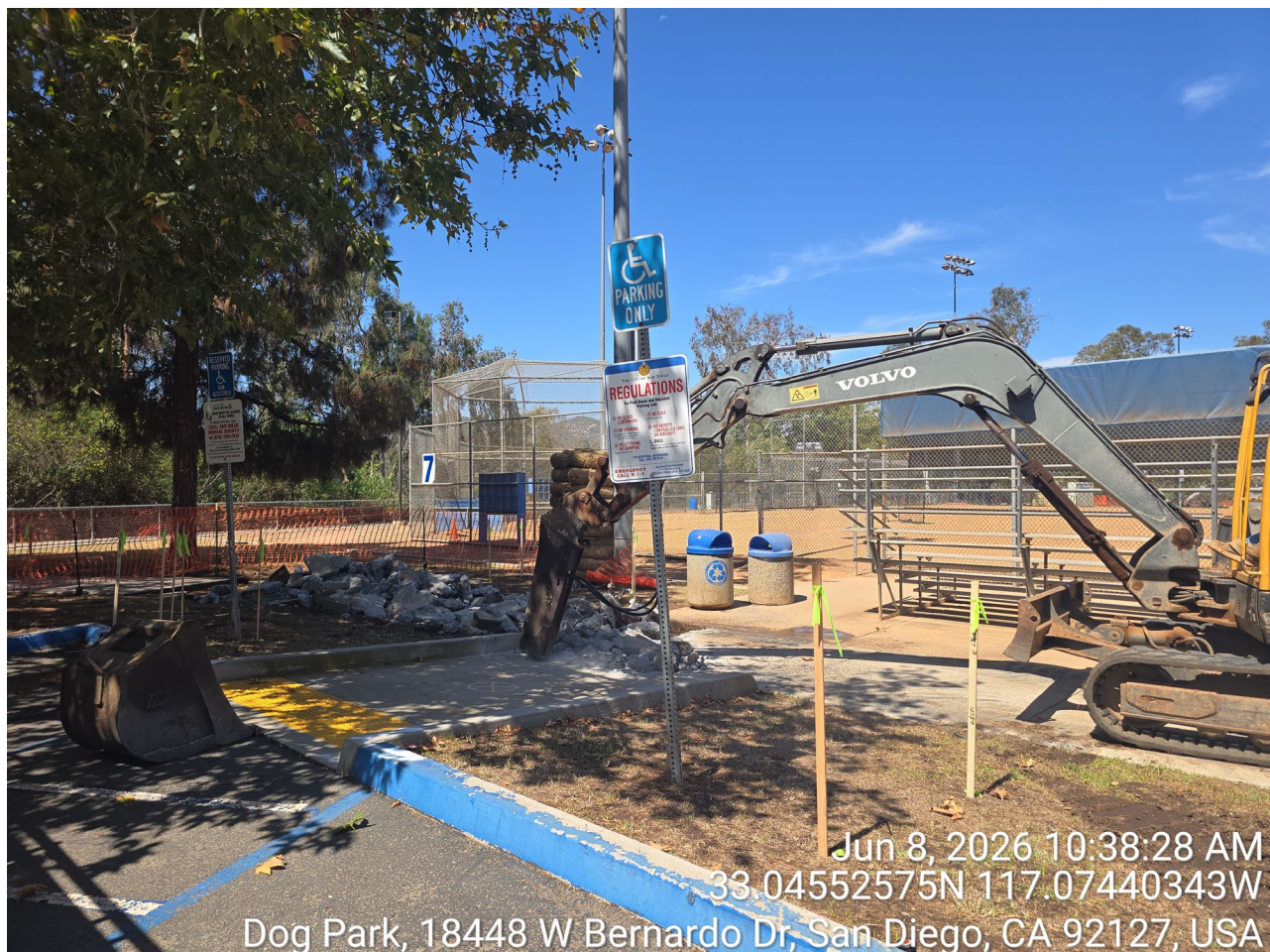
Demolition behind Field 7.
