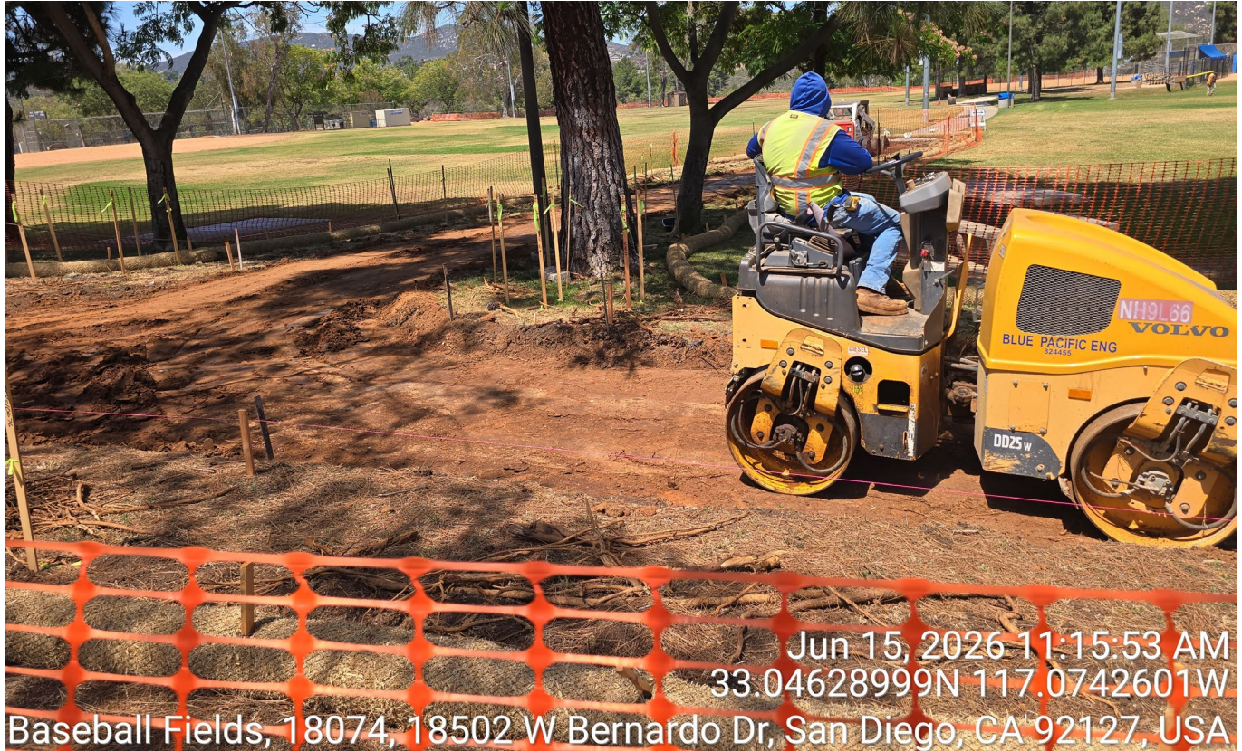
Grading at the north-east of Field 7.
