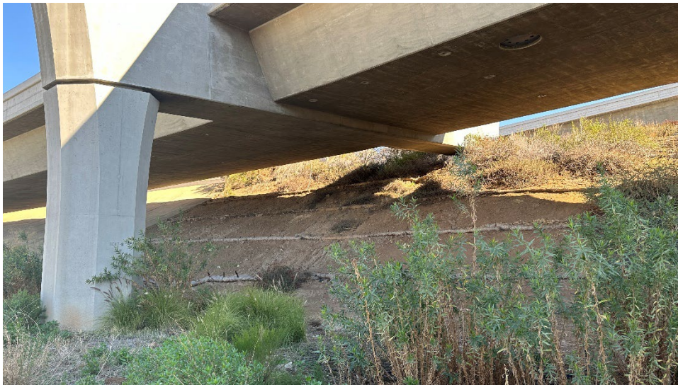
Figure 8. 280+76, Inaccessible (Safety) Area, facing east.
