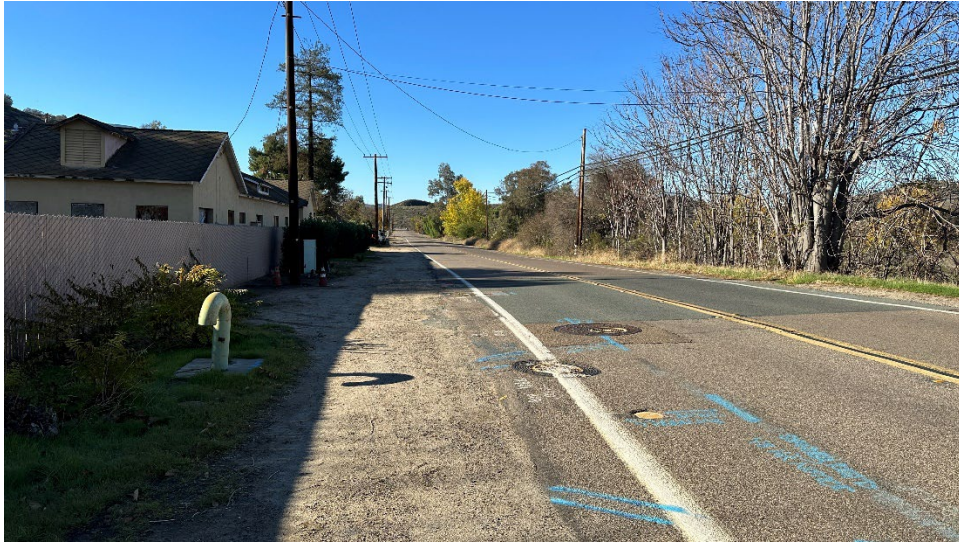
Figure 1. 0+00-4+00, Overview of APE, facing northeast.
