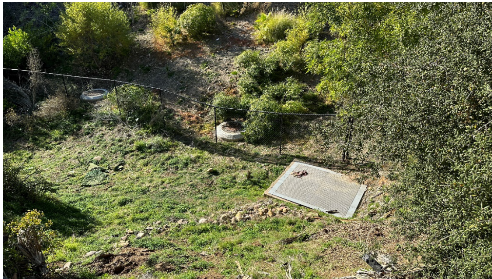
Figure 20. 632+33, Overview of BO Improvement, facing west.
