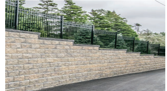
Example Photo of Iron Fence Theme Wall
