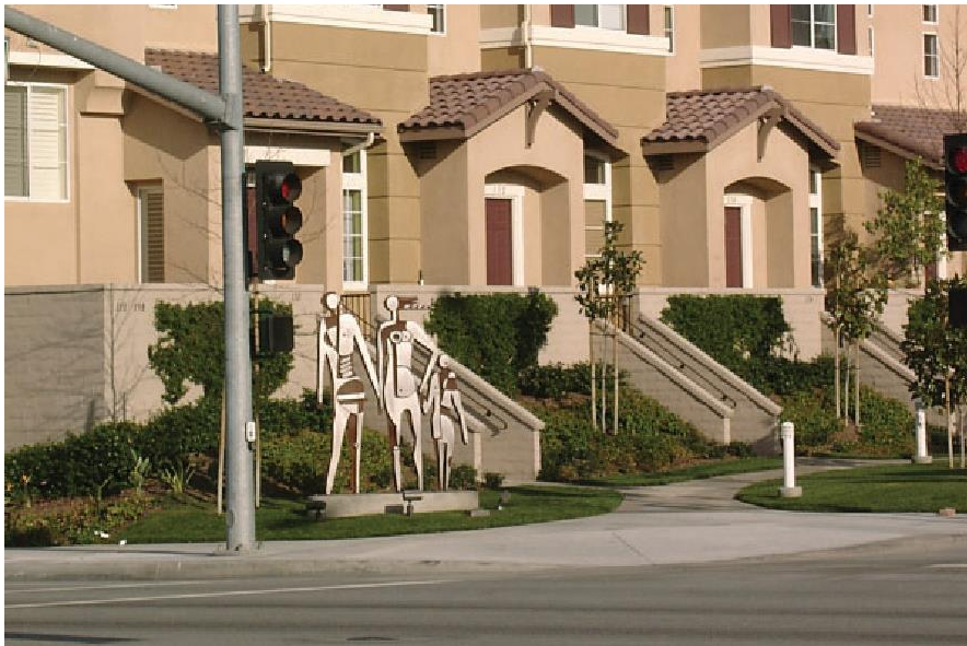
Example photos of building frontage and access.
