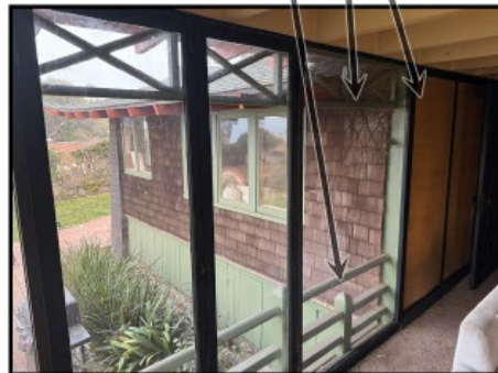
2024 View of the Central Porch and Enclosed Easterly Porch, Facing East
