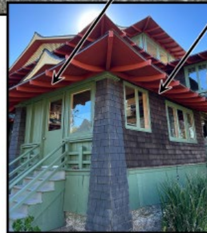
2024 View of the Easterly Enclosed Porch, Facing South
