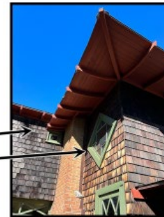
2024 View of the Windows on the Southwest Façade, Facing North
