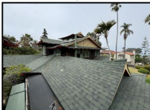
2024 View of the Third Floor of the Residence, Facing West
