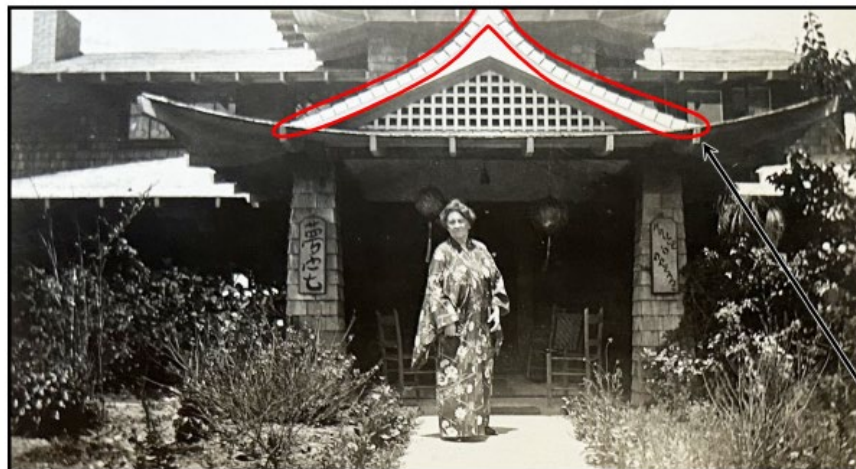
Circa 1911 to 1921 View of Mrs. Howard in Front of the Primary Façade Entrance, Facing Northwest
