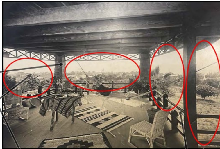
1917 View of the Central Porch, Facing West (Photograph courtesy of Beverly Helm)
