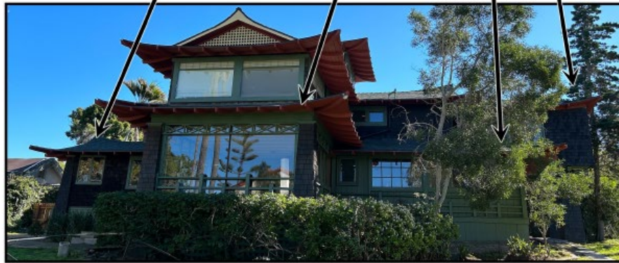
2024 View of the Northwest Façade of the Residence, Facing East
