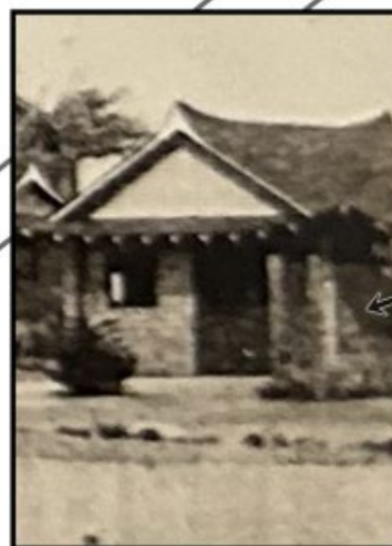
Circa 1921 View of the Primary Façade of the Detached Garage, Facing West
