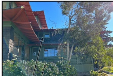
2024 View of the Westerly Enclosed Porch, Facing Southeast
