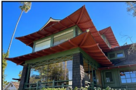
2024 View of the Central Enclosed Porch, Facing East
