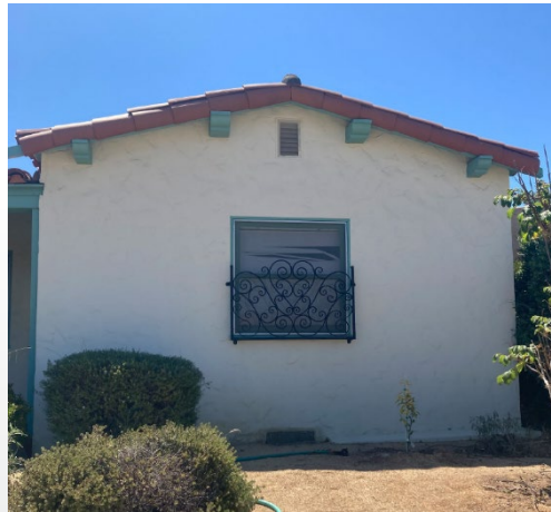
Fascia board under low-pitch, gabled roof with tile raked over edge
