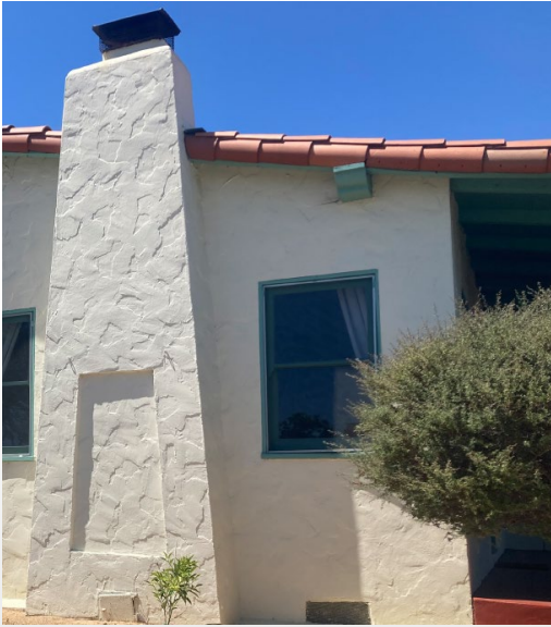
Hand-trowelled stucco cladding
