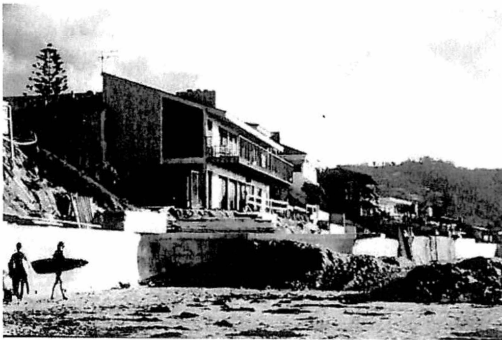
Photo #7: 1979 view at 8516 El Paseo Grande with new seawall constructed (Kuhn, 1984)
