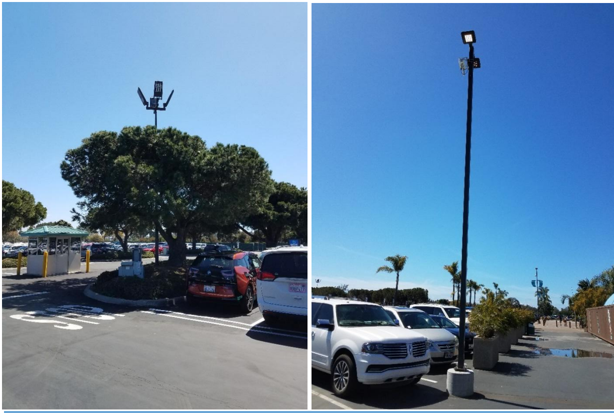
Typical parking lot lighting
