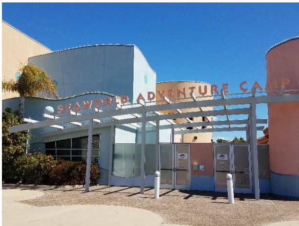
View of SeaWorld Adventure Camp building from Perez Cove Way
