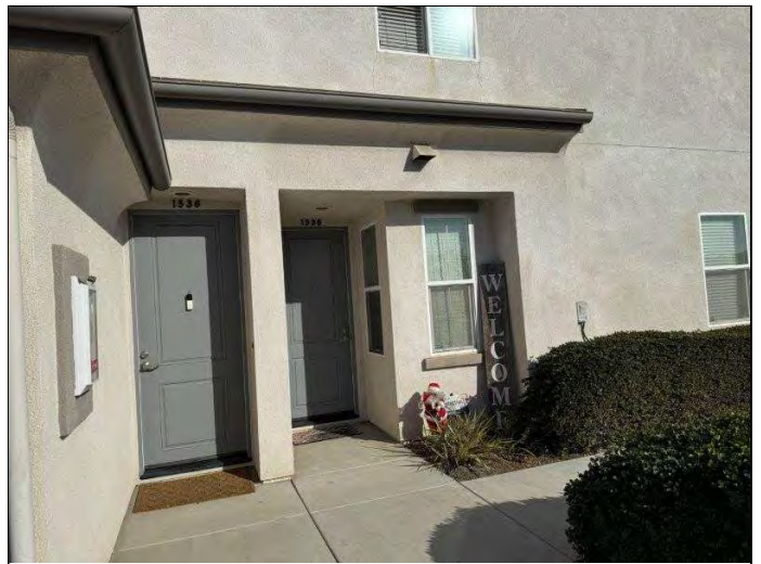
10. Unit entrance doors on south side to 1536 and 1540.
