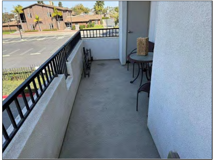
14. Balcony at unit 1554.
