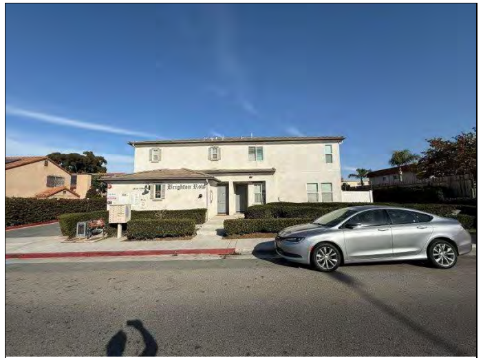
4. View of subject property from right of way.
