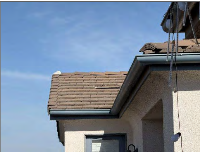
15. Typical concrete roof tile and gutter system.
