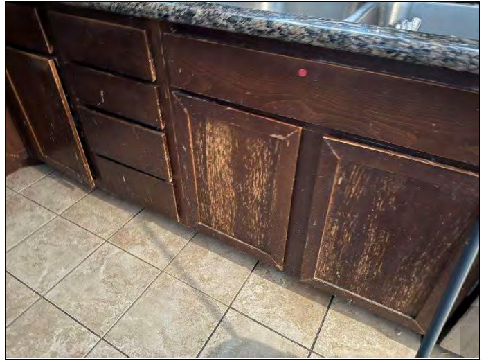
38. Kitchen cabinet finish at sink in unit 1540.
