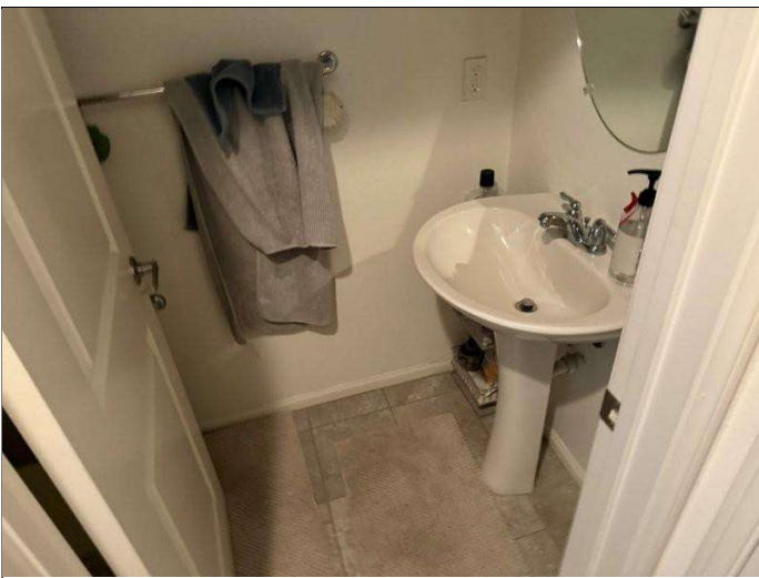
47. Bathroom at unit 1546.
