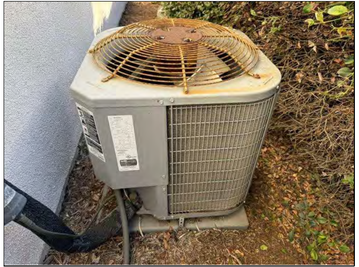
26. Typical split system condensing unit.
