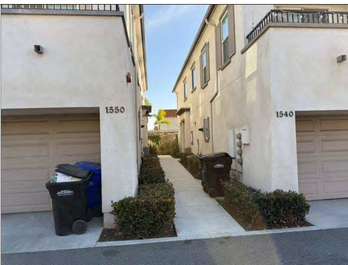
17. View between 1546, 1548, 1550 Building and 1540, 1538, 1536 Building.
