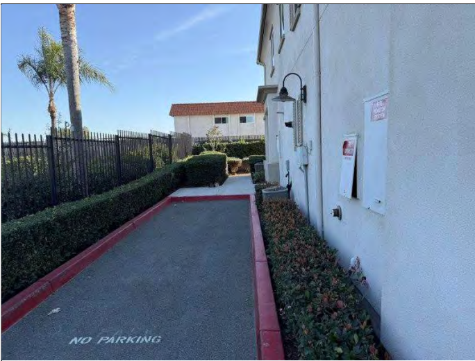
9. North side of site view to the east.
