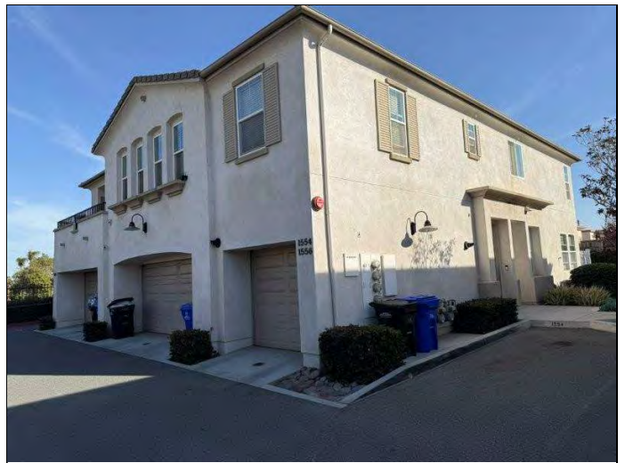
16. View to 1554, 1556, and 1558 building.
