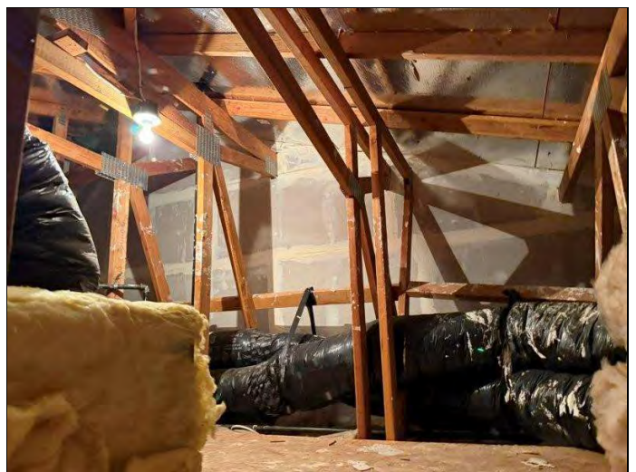
18. Attic space with partition drywall between units, unit 1556 shown.
