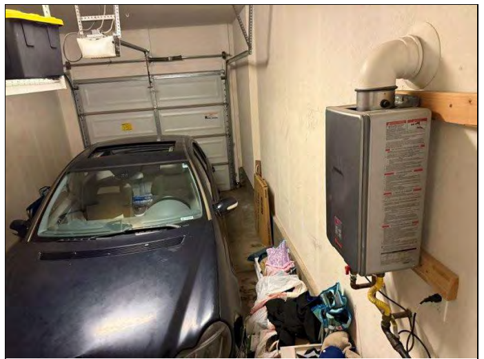
48. Garage at unit 1546.
