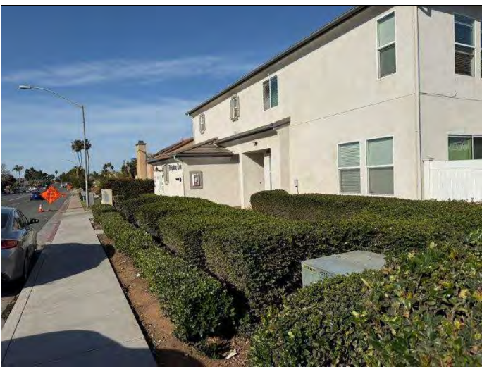
5. View west along south side of site.
