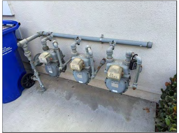
20. Typical individual gas service meters.
