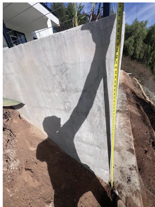
SOUTHWEST WALL CORNER
