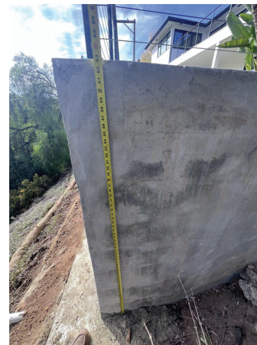
SOUTHEAST WALL CORNER
