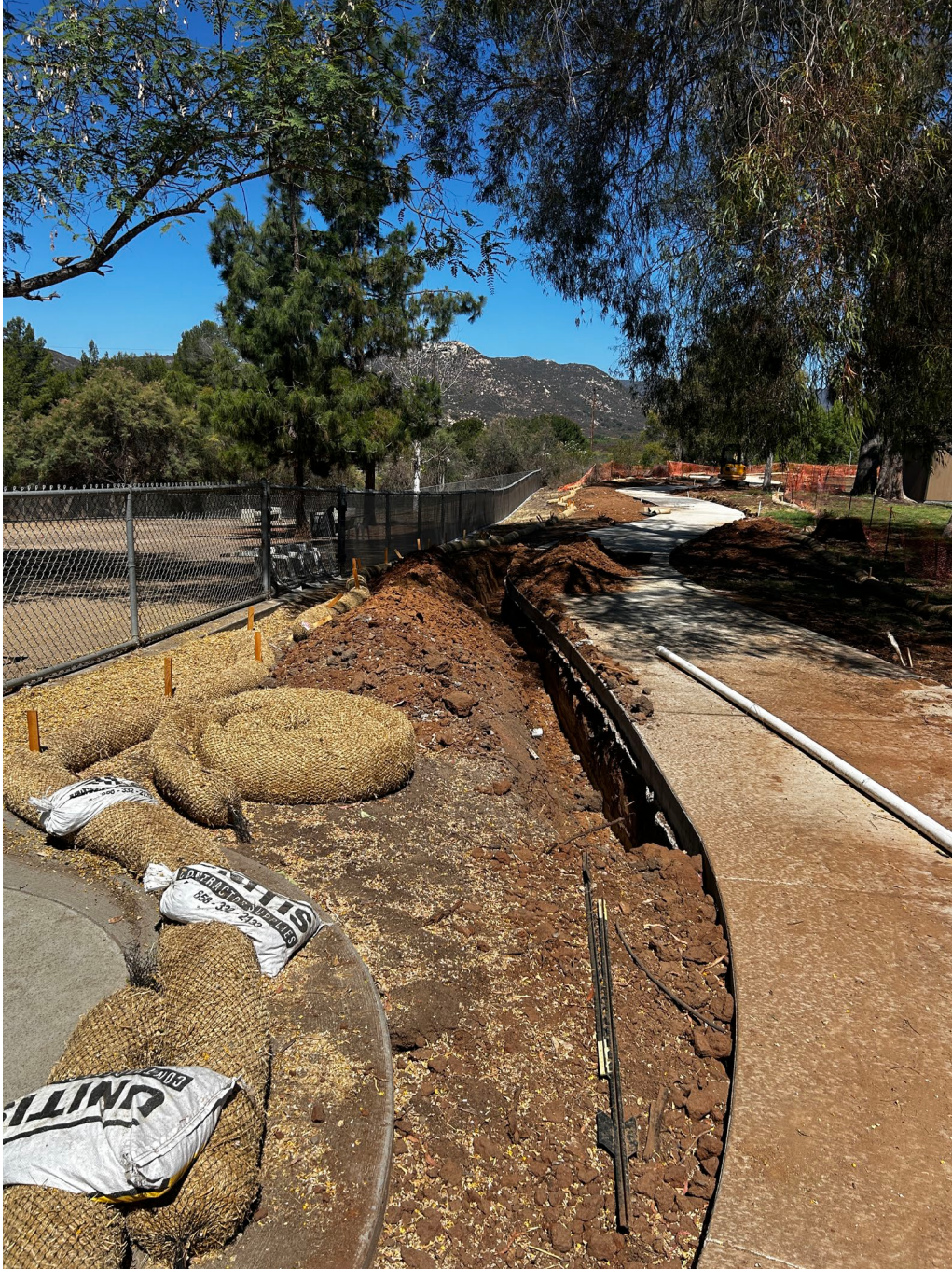
New walkway from the dog park to parking lot at Field 8
