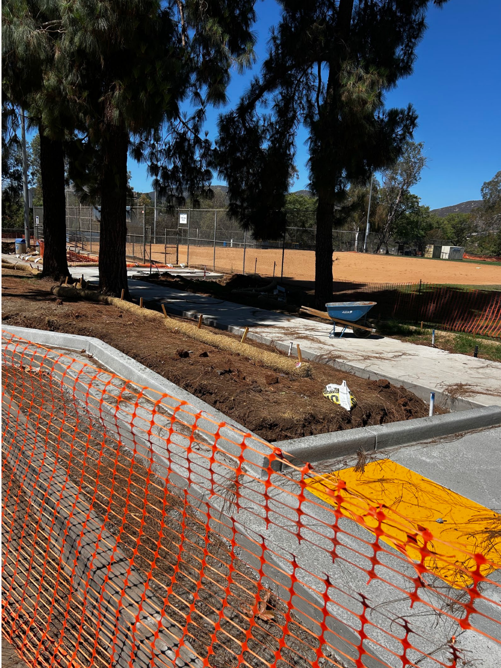
Improvements to the walkway adjacent to parking lot at Field 7
