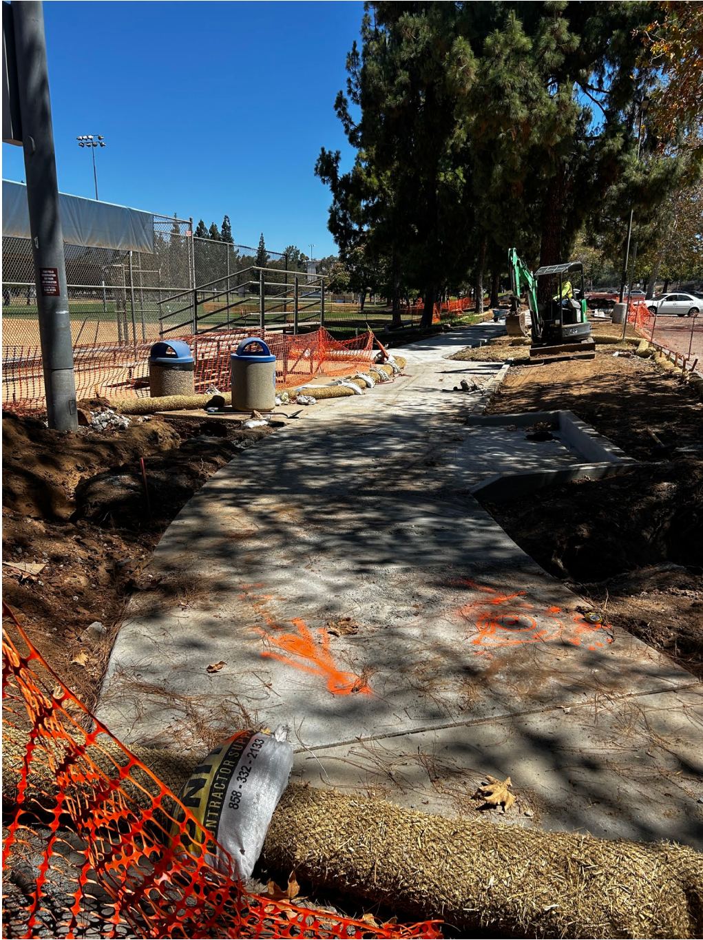
Walkway improvements from Field 5 to Field 7
