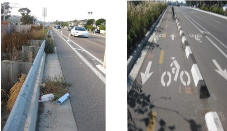
Left: Morena Blvd Class IV Cycle Track is overgrown with tumbleweeds and dirty with gravel, trash, and broken bollards. Right: The Friars Road Cycle Track seems to be undergoing renovations.
