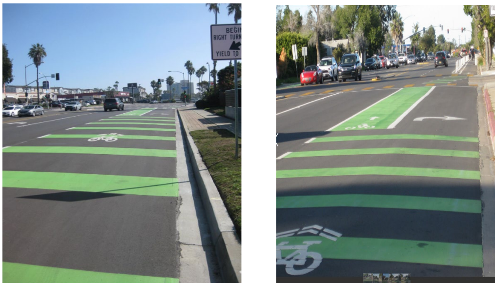
Left: Conflict striping that leads to a bike box on (I Heart) Clairemont Drive. Right: Bike box provides enhanced visibility.
