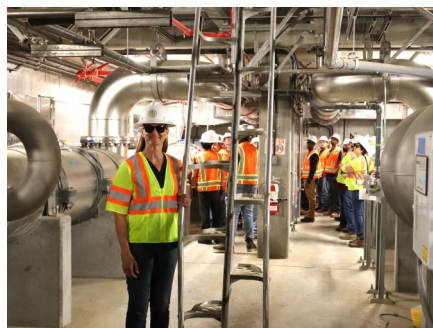
City of San Diego Project Visit 03/25/2026
