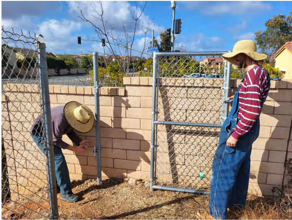
Photo 18. City staff performing gate installation.
