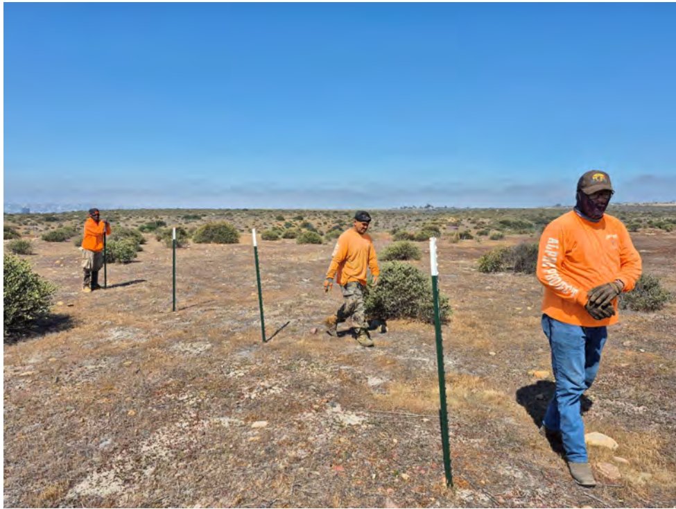
Photo 82. Contracted crew performing fence installation.
