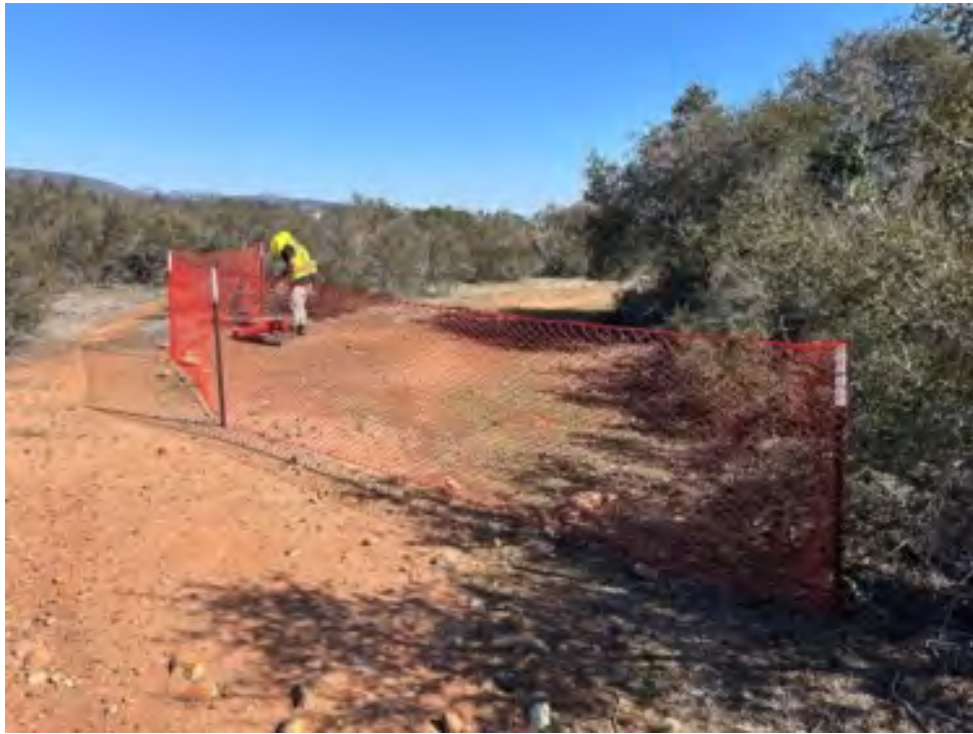
Photo 22. Contracted crew performing fence installation.
