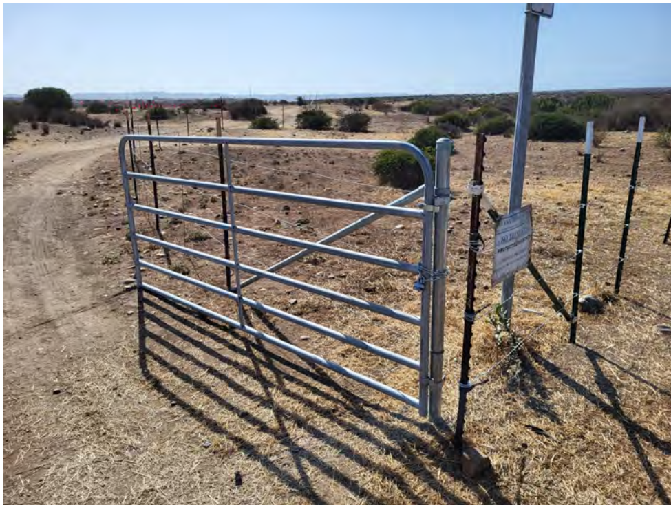
Photo 83. City staff performed gate installation.
