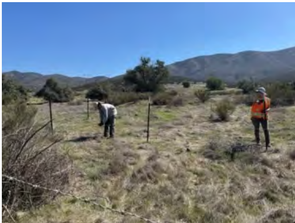
Photo 60. Contracted crew performing fence installation.
