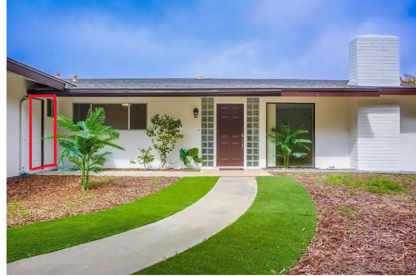
FRONT ELEVATION (ENTRY DOOR)
