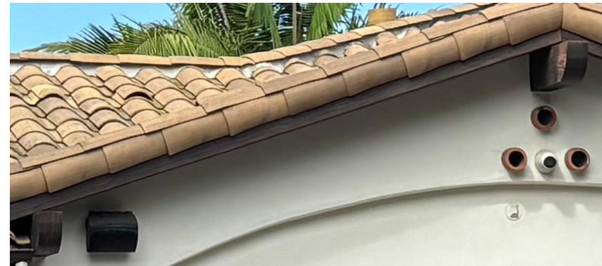
Exposed Wood – to match existing
