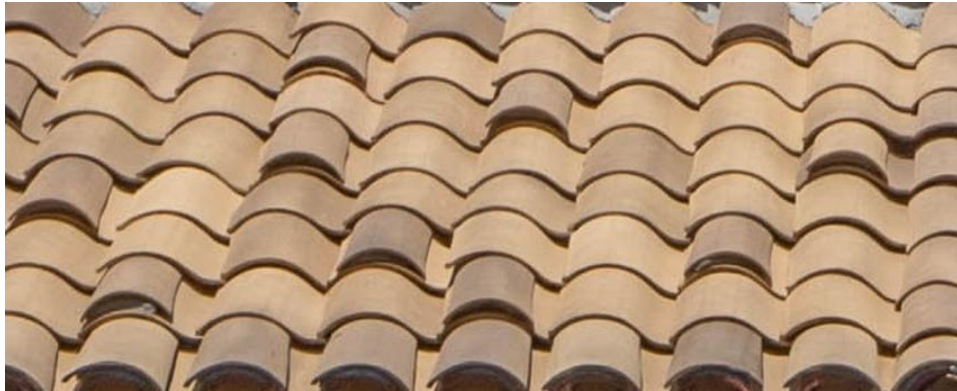
Roof- Spanish tile – to match existing
