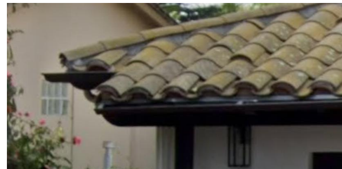
Copper Gutters – to match existing
