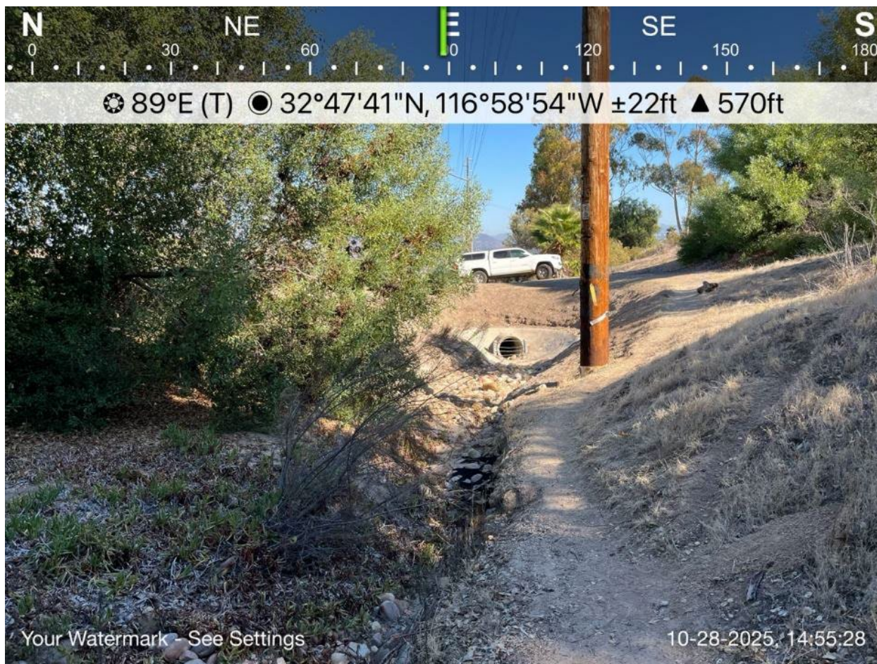
Photo 8. Work Location 439+20, NWW-ALT-04; view of culvert inlet that directs water from both NWW-ALT-04 and -05 into an underground stormwater system of pipes that are assumed to flow 0.75-miles to a channelized reach of Forester Creek; View facing east. October 28, 2025.
