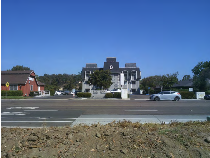
EDR Map ID No. AF186 - Dominion West Office Suites at 4045 Bonita Road. An AT&T Mobility suite is listed as a chemical storage site due to lead-acid batteries. The adjacent American Medical Response at 4035 Bonita Road is also listed as a chemical storage facility. There are no documented leaks or spills from either facility.
