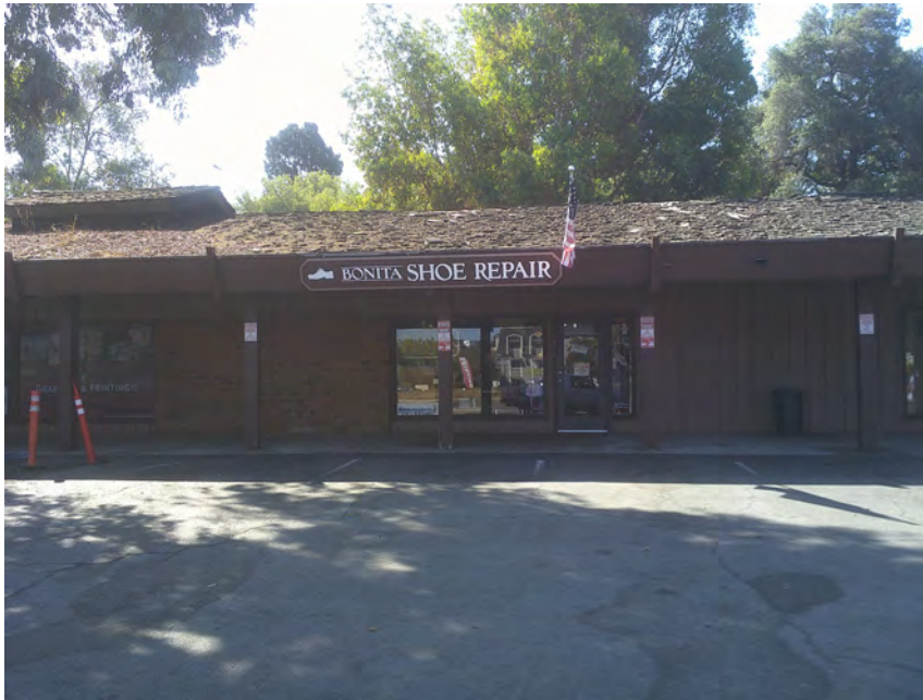
EDR Map ID No. AI188 - Former Bonita Village Cleaners at 4050 Bonita Road. There are no documented leaks or spills from the former cleaners. Site is currently occupied by Bonita Shoe Repair.
