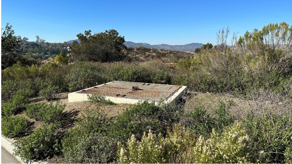
Figure 7. 267+39, Overview of APE, facing west.
