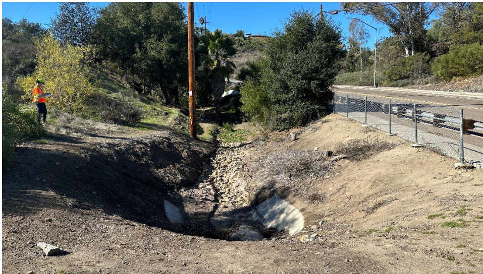
Figure 12. 439+37, Overview of Grossmont Tunnel Access, facing west.
