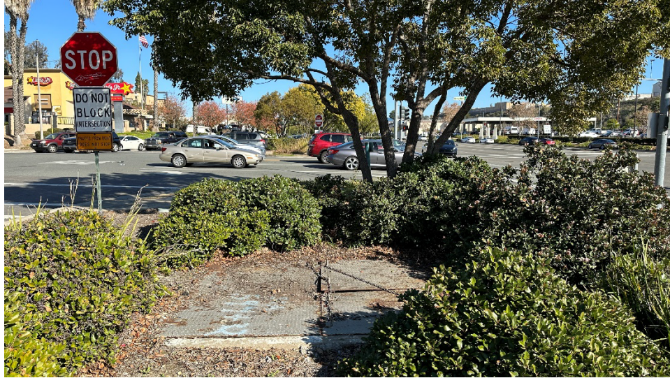
Figure 17. 594+32, Overview of BO Improvement, facing northeast.
