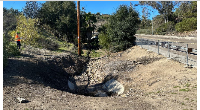
Photo 6. Grossmont Tunnel access overview. View facing west.
