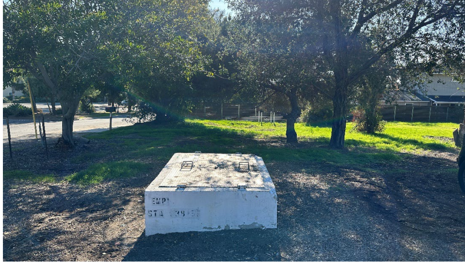
Figure 21. 638+59, Overview of AV Improvement, facing south.
