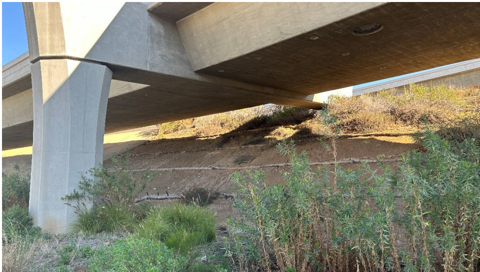
Figure 8. 280+76, Inaccessible (Safety) Area, facing east.
