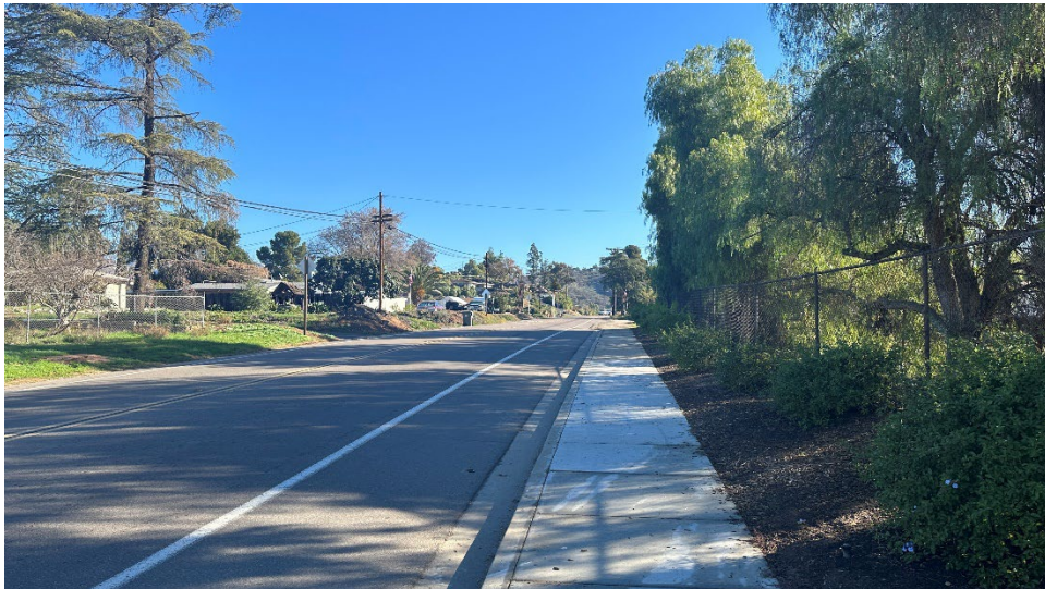
Figure 2. 64+75, Overview of APE, facing northwest.
