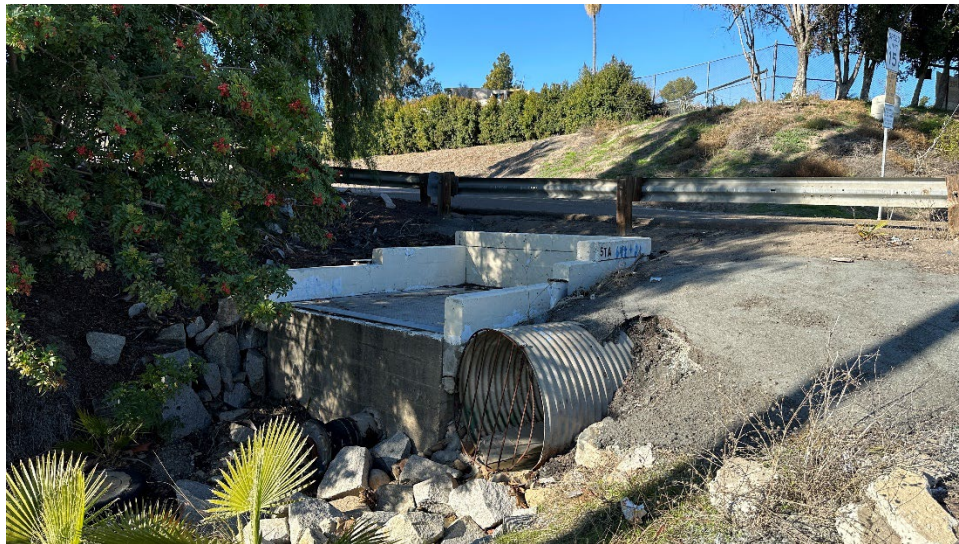
Figure 22. 644+21, Overview of BO Improvement, facing northwest.
