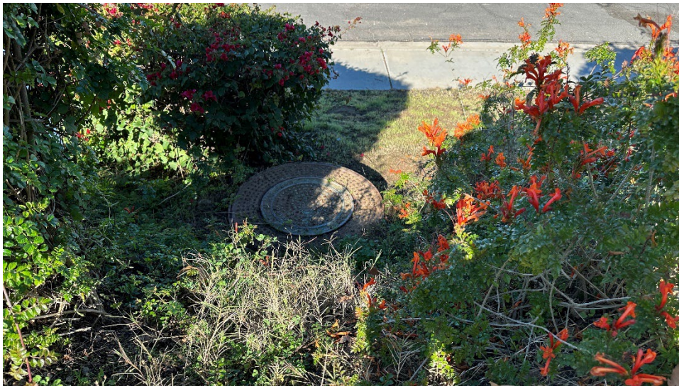
Figure 4. 220+85, Overview of Manhole within Residential Landscape, facing northwest.
