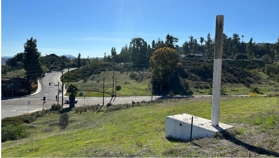
Figure 11. 434+62, Overview of Valve Location, Increasing in Height, facing south.
