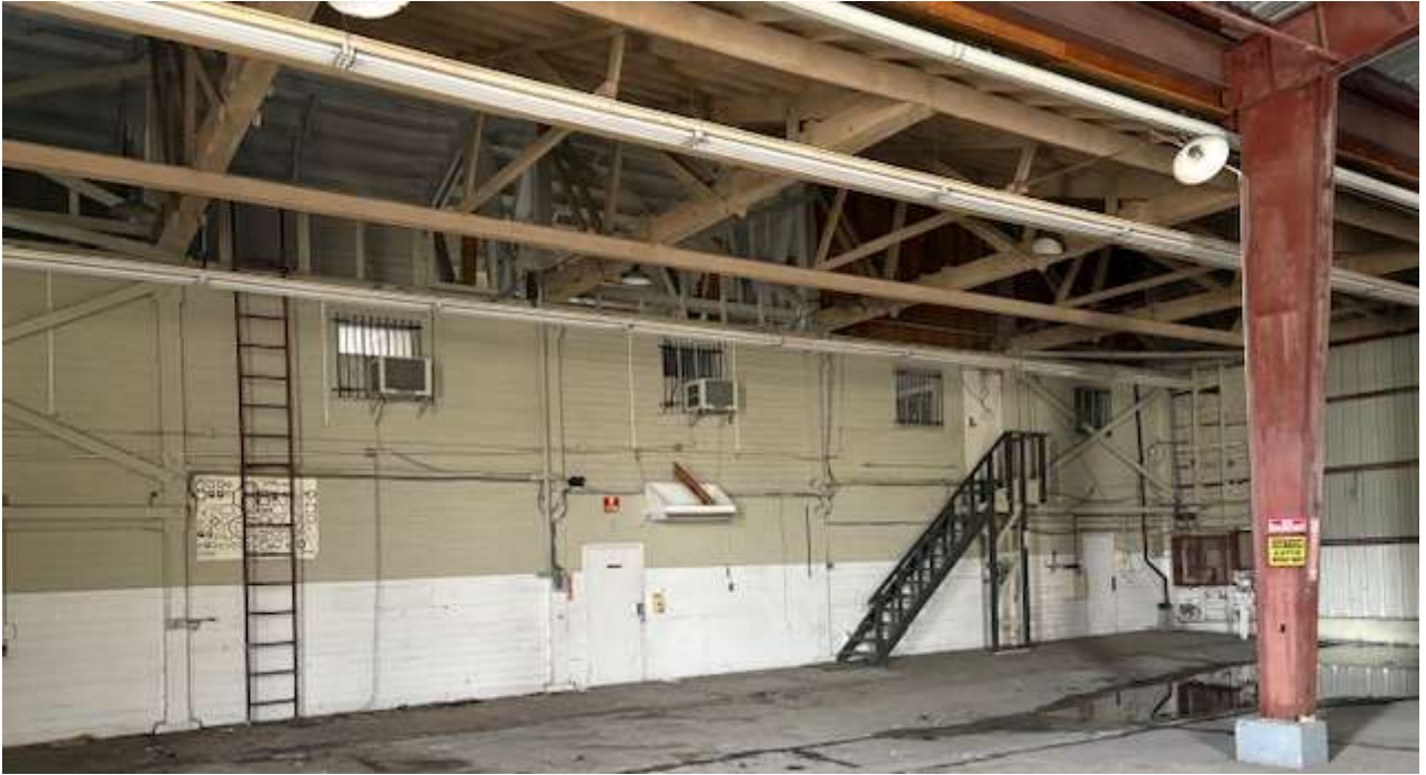
Interior Large Hangar/Office Alternate Entrance
