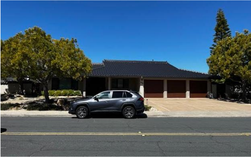
5. West elevation taken from across the street.
