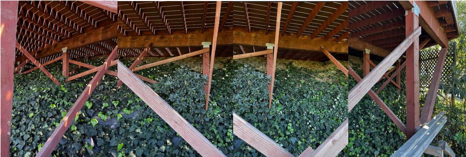
8. Panoramic view of underside of backyard deck
