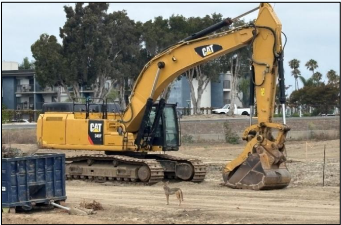
Coyote near construction equipment. Photo Credit: Jayne Romero
