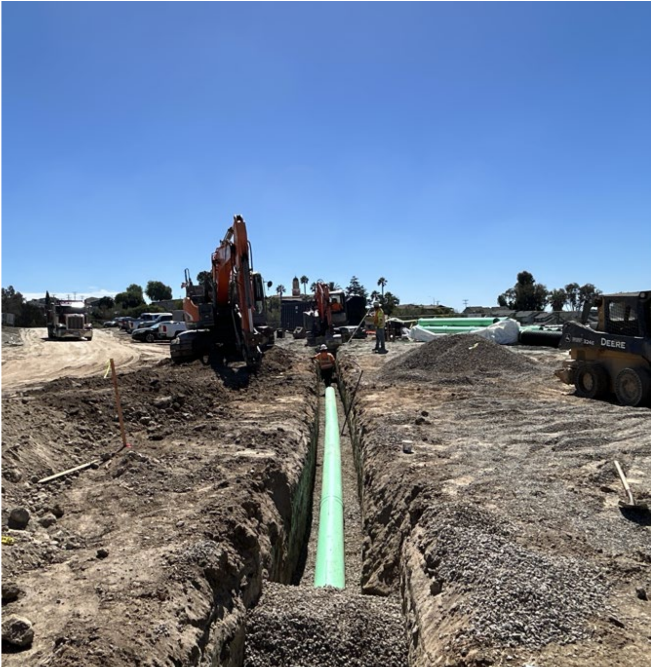
Storm drain installation
