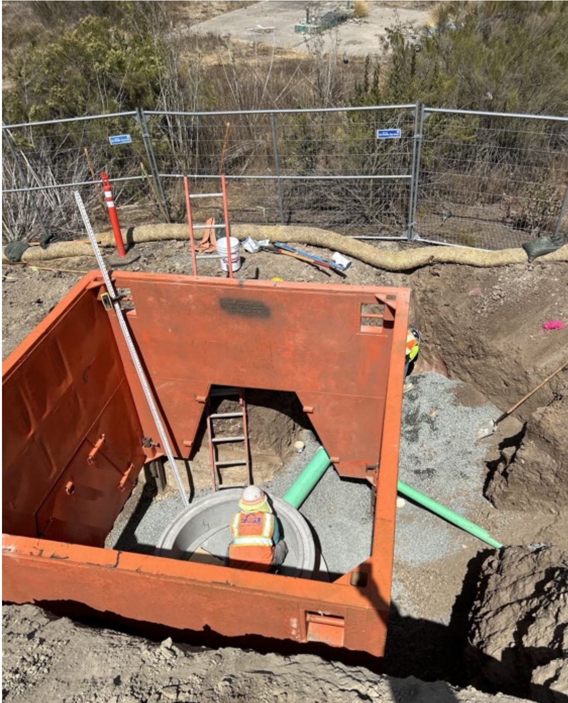
Sewer main extension and lateral connection
