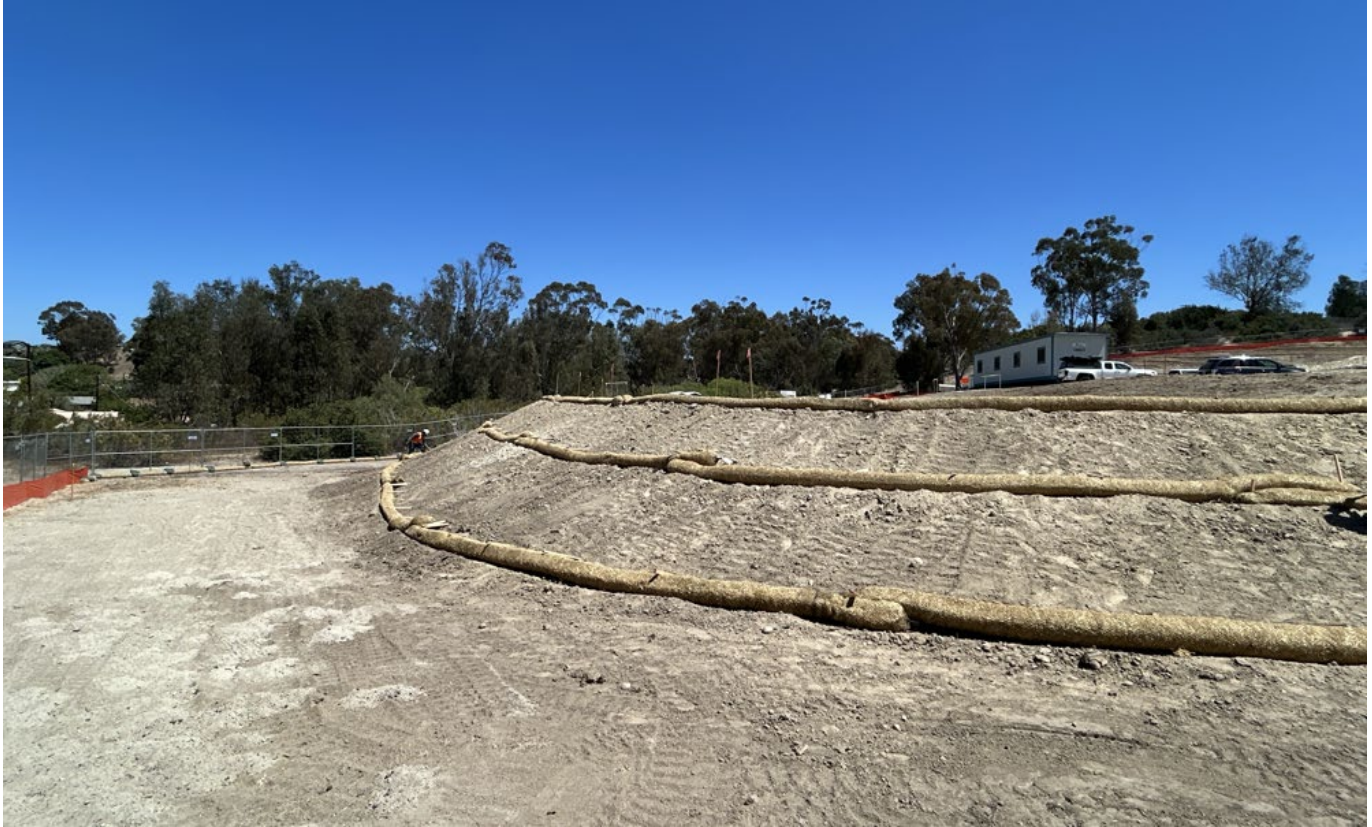
Installation of BMP's on inactive slopes
