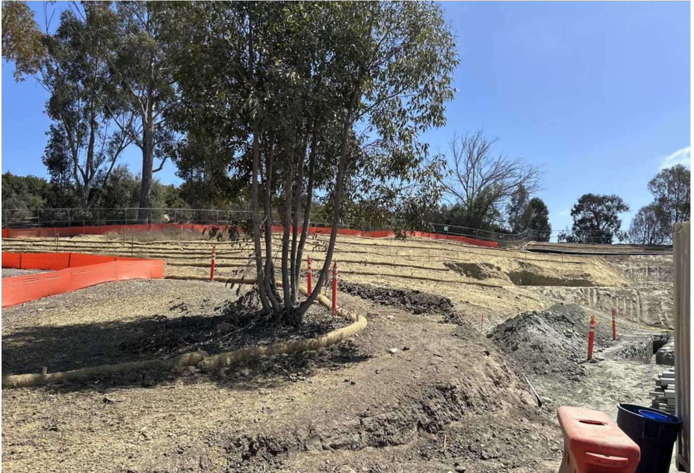
Inactive slopes stabilized with fiber rolls and soil binder
