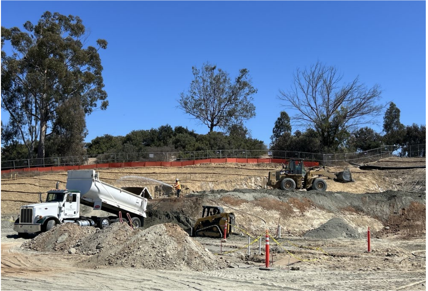
Import fill material and build up grade at upper level building pad.
