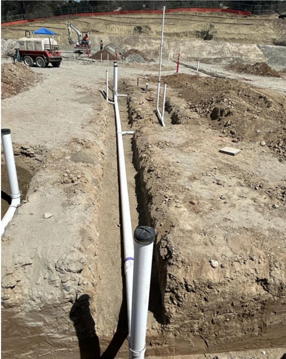
Installation of under-slab drain pipes
