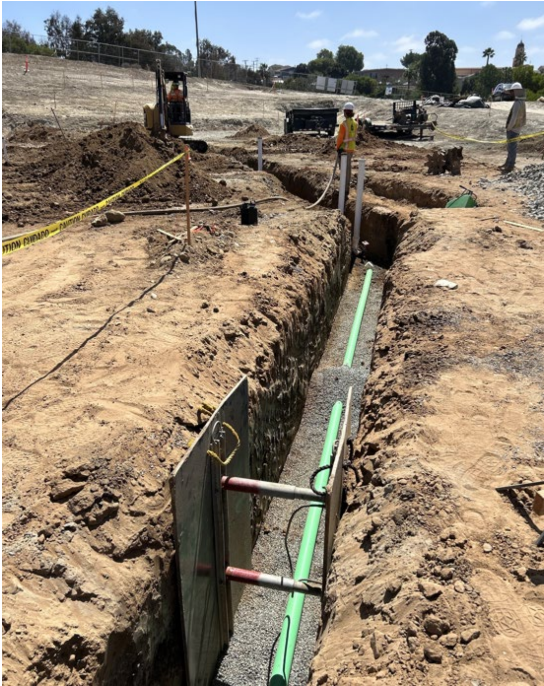
Installation of sewer lateral to building pad
