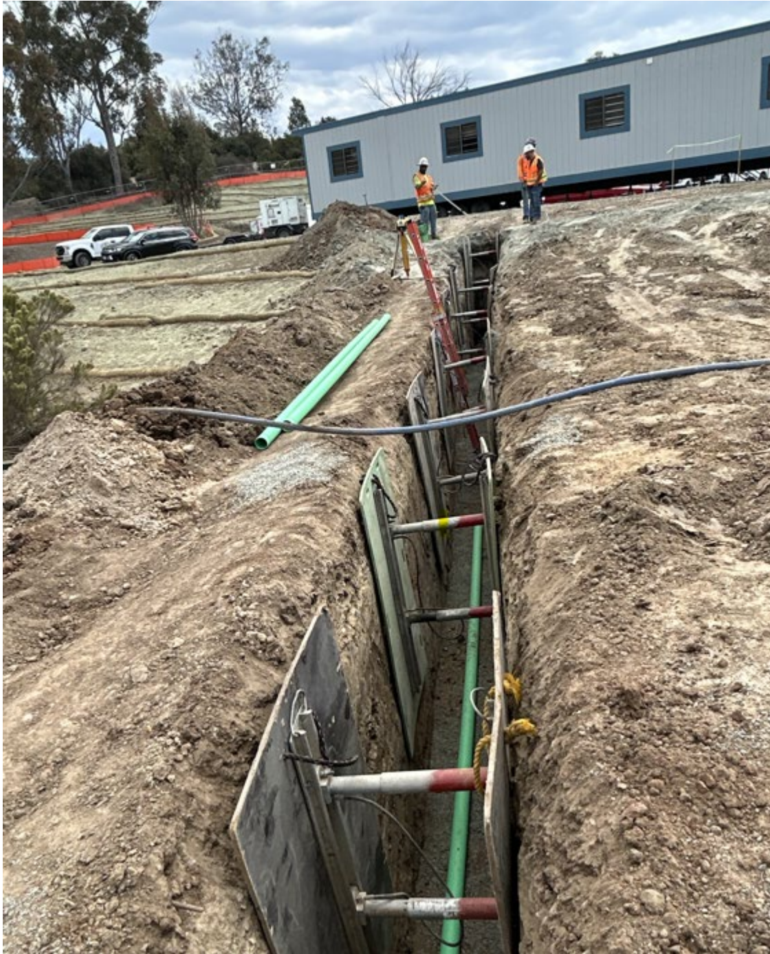
Installation of sewer lateral
