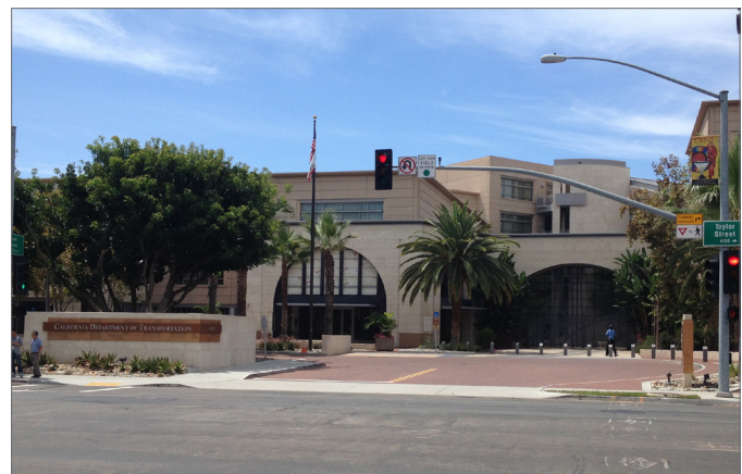
The Caltrans District 11 Headquarters institutional use occupies the largest site in the Taylor Sub-District.
