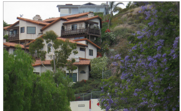
This multi-family development in the Linwood Sub-District is a good example of using building articulation, altitoo roof effect, and creative site design to integrate with the topography and achieve a human-scale appearance.
