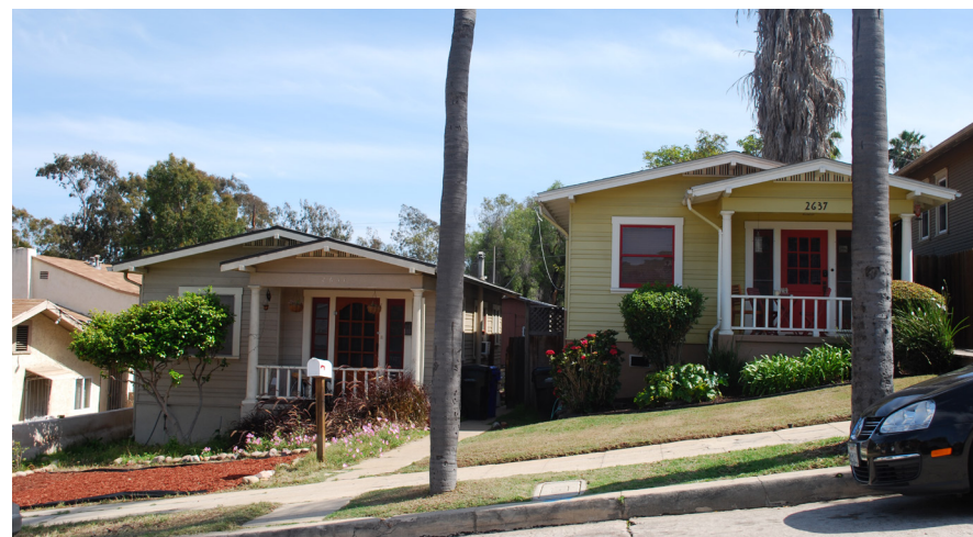
Raised foundations are a response to sloping topography that minimizes grading.
