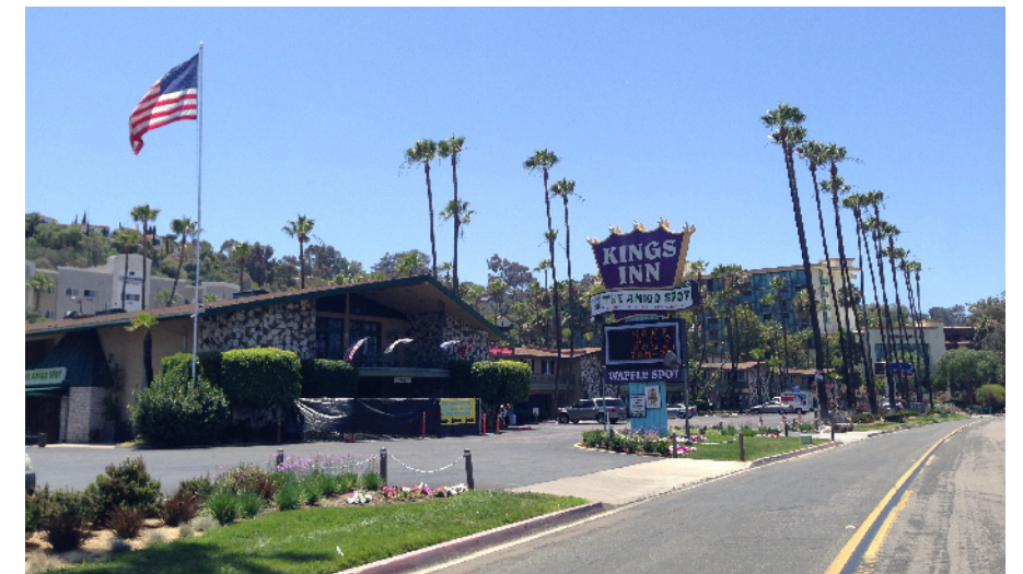
Properties such as King's Inn, built in 1959, may now potentially be eligible for listing as a historic resource.
