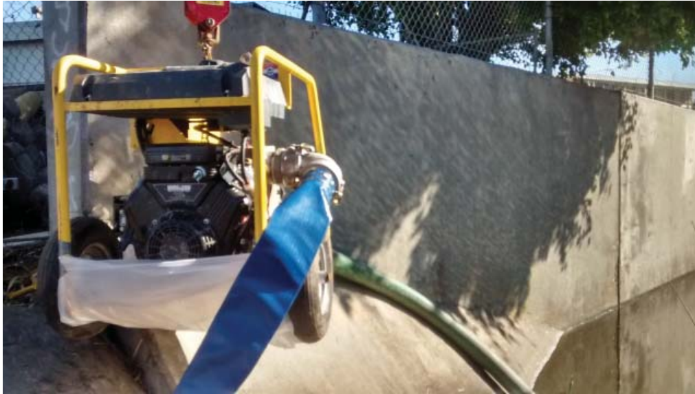
Bypass pump hung above channel. February 5, 2016
