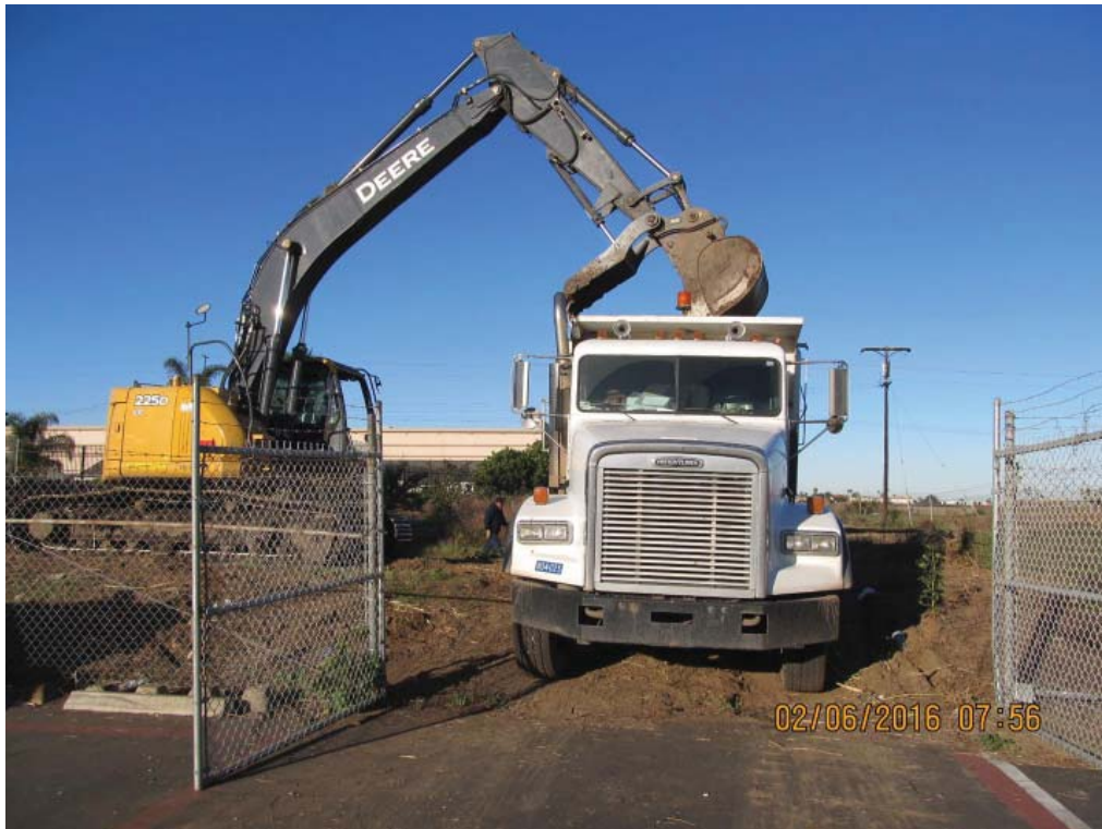
Debris loading into dump truck for removal from site. February 6, 2016
