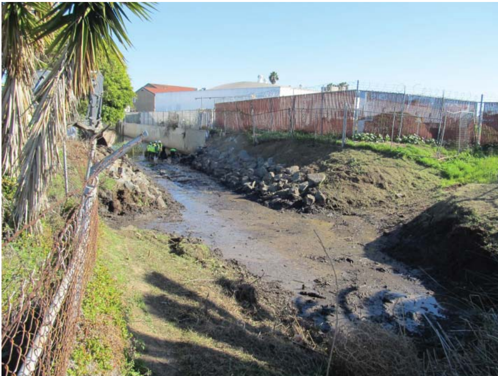
Excavator clearing channel (facing south). February 5, 2016
