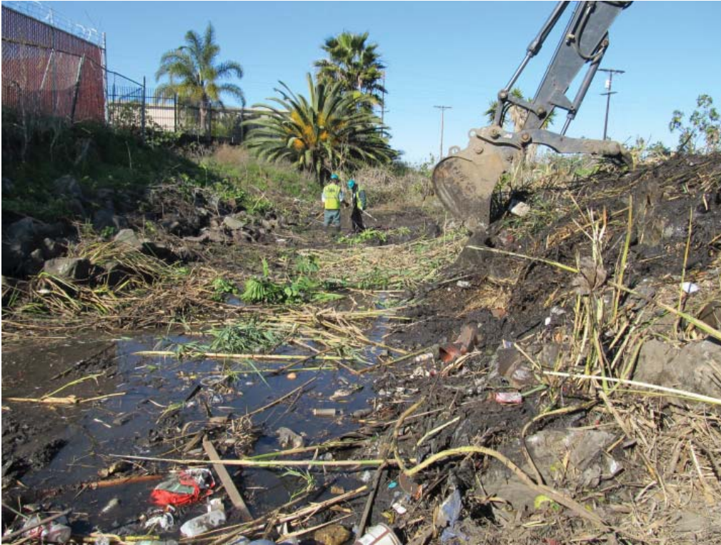
Excavator clearing channel (facing north). February 5, 2016
