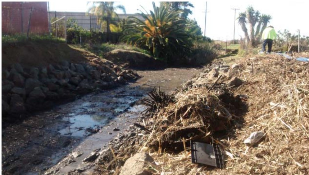
Cleared channel (facing north). February 5, 2016
