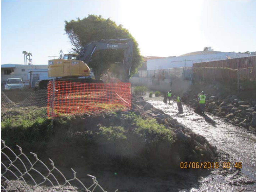
Removal of trash and vegetation from within the channel using hand-held tools. February 6, 2016
