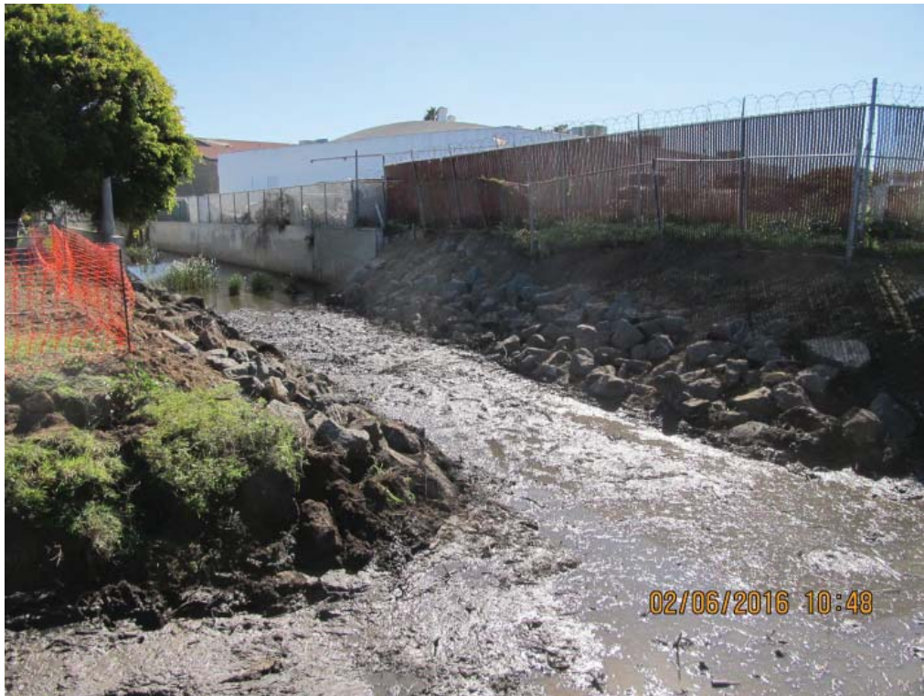
Cleared channel (facing south). February 6, 2016
