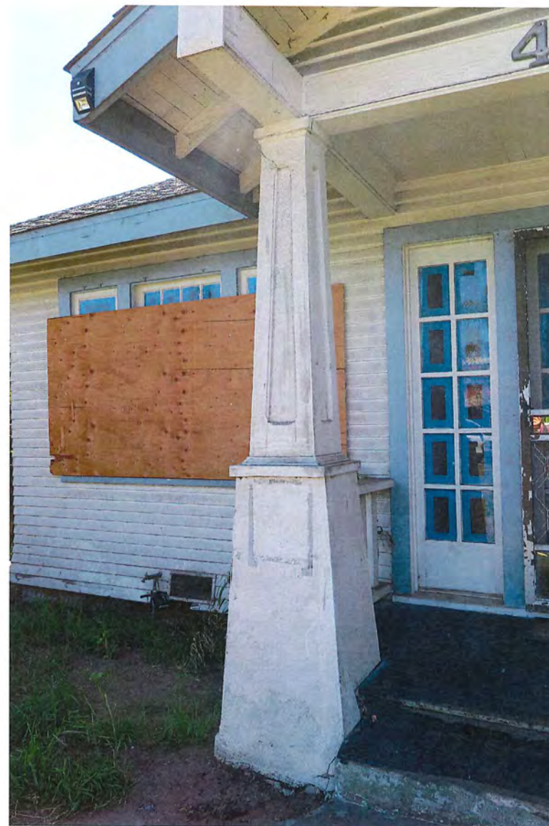
Plate 4: Close-up of a tapered column, plinth, and base on the north façade.
