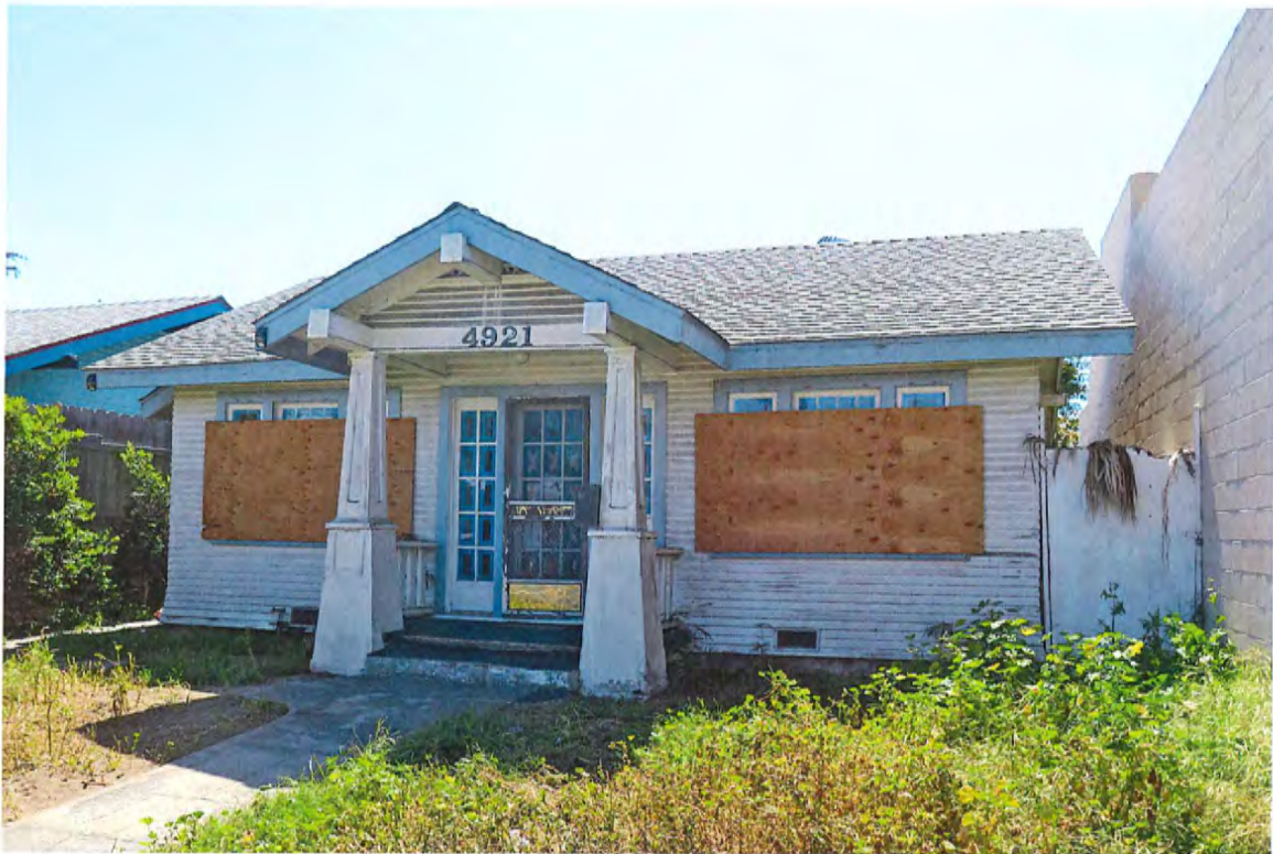
Plate 1: View of the north façade. Note the sloping foundation visible on the leftmost corner.
