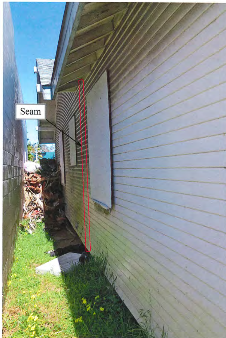
Plate 5: View of the west façade showing the remodel seam between the original structure and the 1947 addition.
