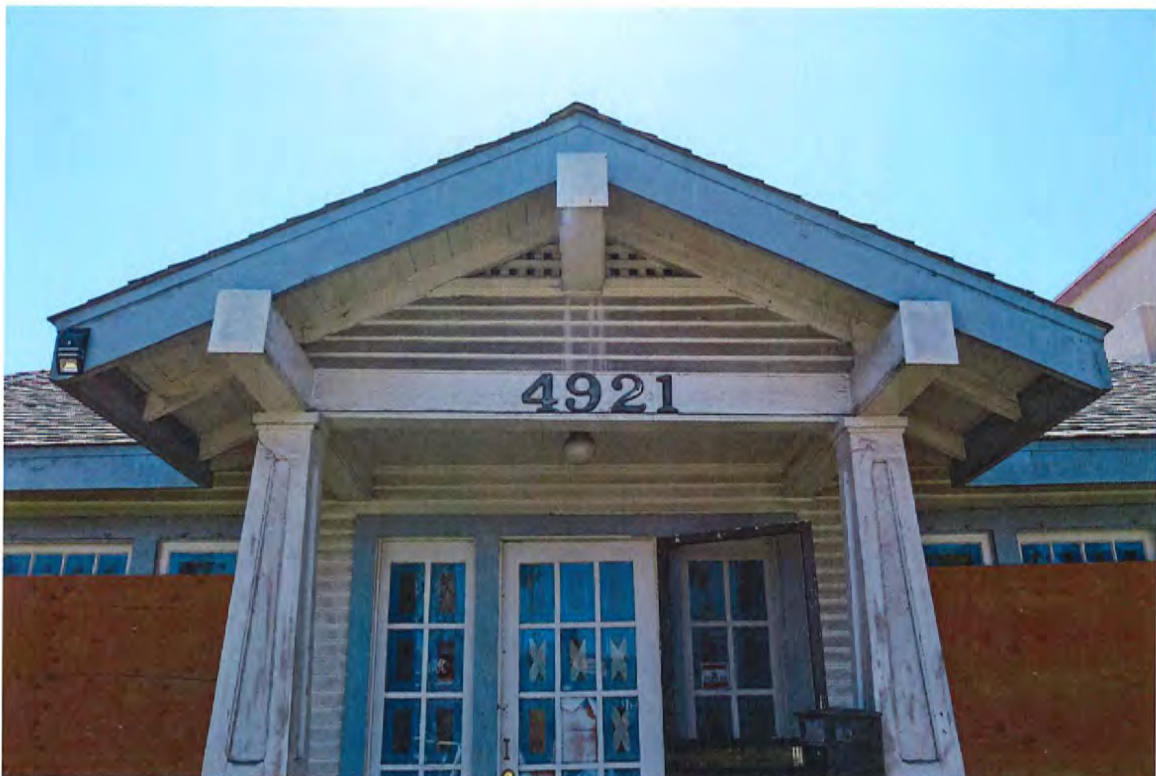
Plate 2: View of the north façade showing the porch's tapered columns and gabled pediment.
