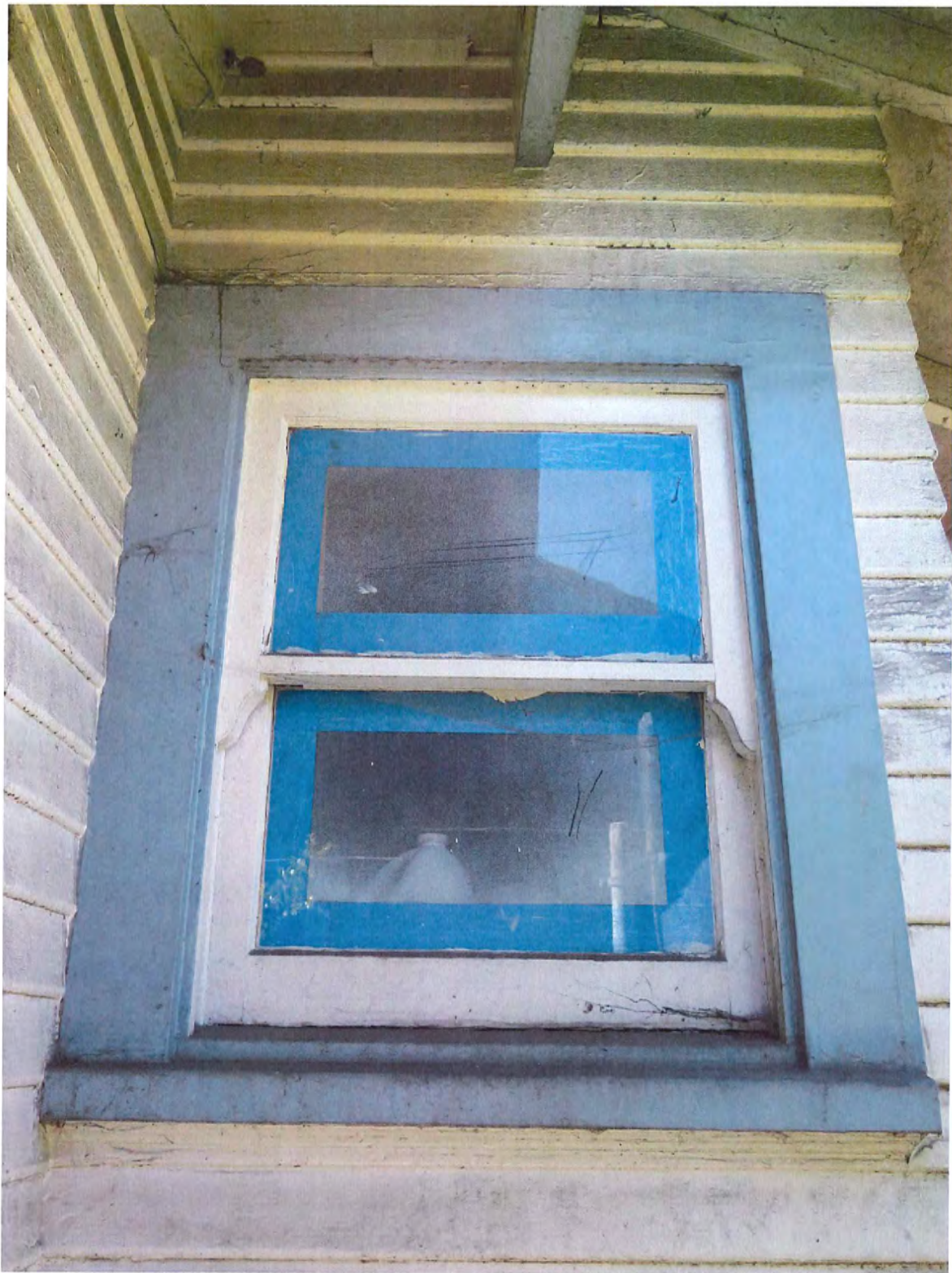
Plate 14: Close-up of an original, wood-framed, double hung window on the east façade.
