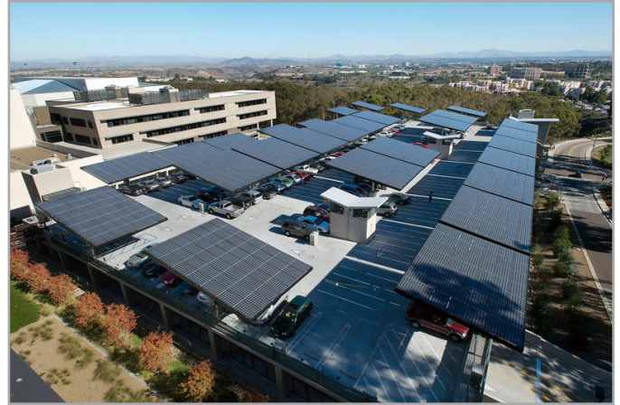
Opportunities exist for the installation of photo-voltaic systems atop the flat roofs of many businesses in North Park's business districts.
