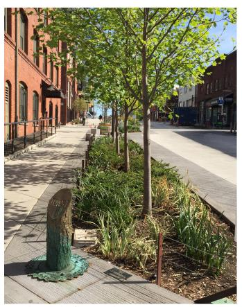
Bioswales and other filtrating techniques can serve the dual function of creating aesthetically pleasing urban areas and treating stormwater.
