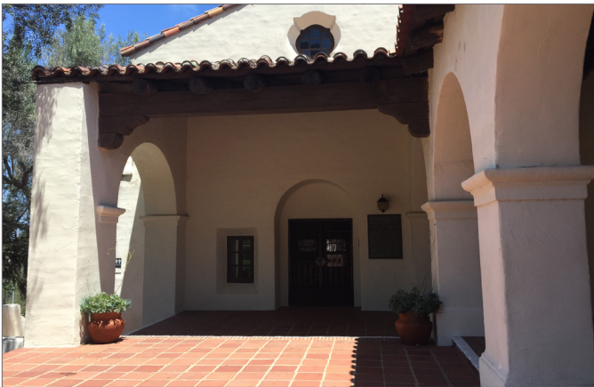
Thick building walls, tile roofs, and shade-providing porticos are pre-1871 building elements that reduce solar heat gain and energy use.
