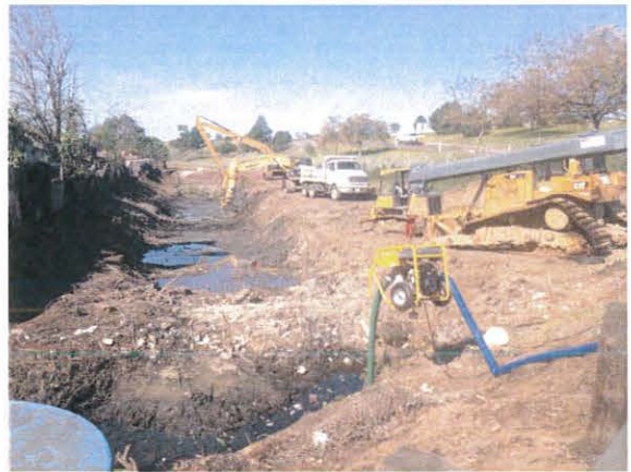
Photograph 8: Looking west into the channel from the east end of the project area at maintenance work and upstream pumping, which was initiated to clear flows coming from upstream of the project area (MMP Map 130; Figure 3).
