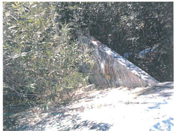
Photograph 6: Looking at one of the three concrete energy dissipators installed along the north end of the channel (MMP Map 130; Figure 3).
