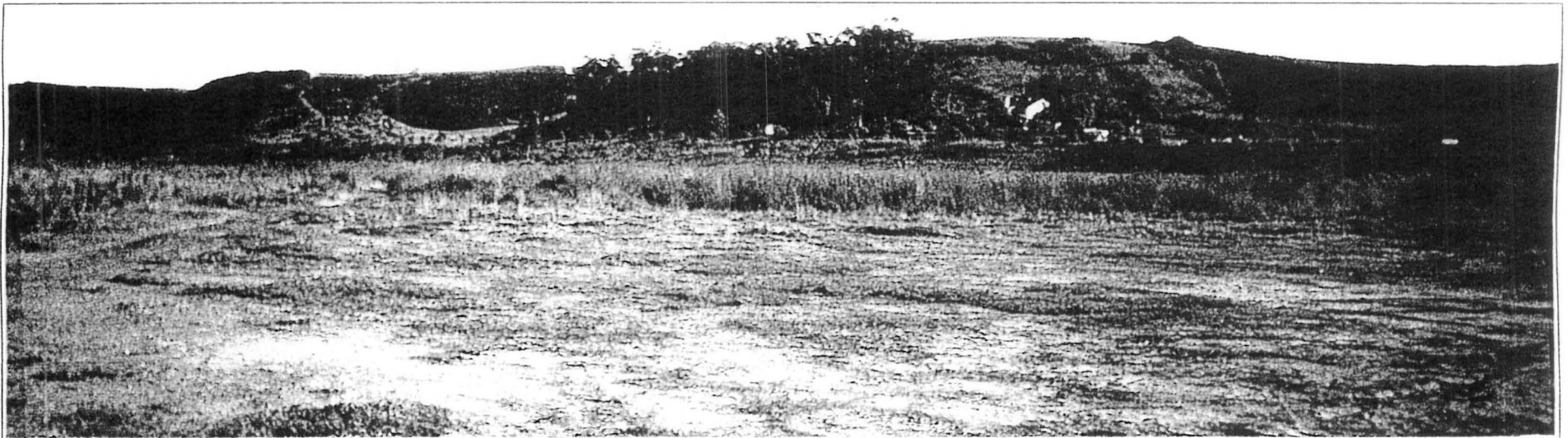
H. View of project site from the San Dieguito River Valley.
