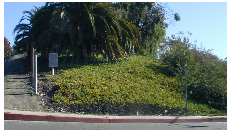
A landscaped berm is used here to provide physical separation at an interchange with State Route 94.
