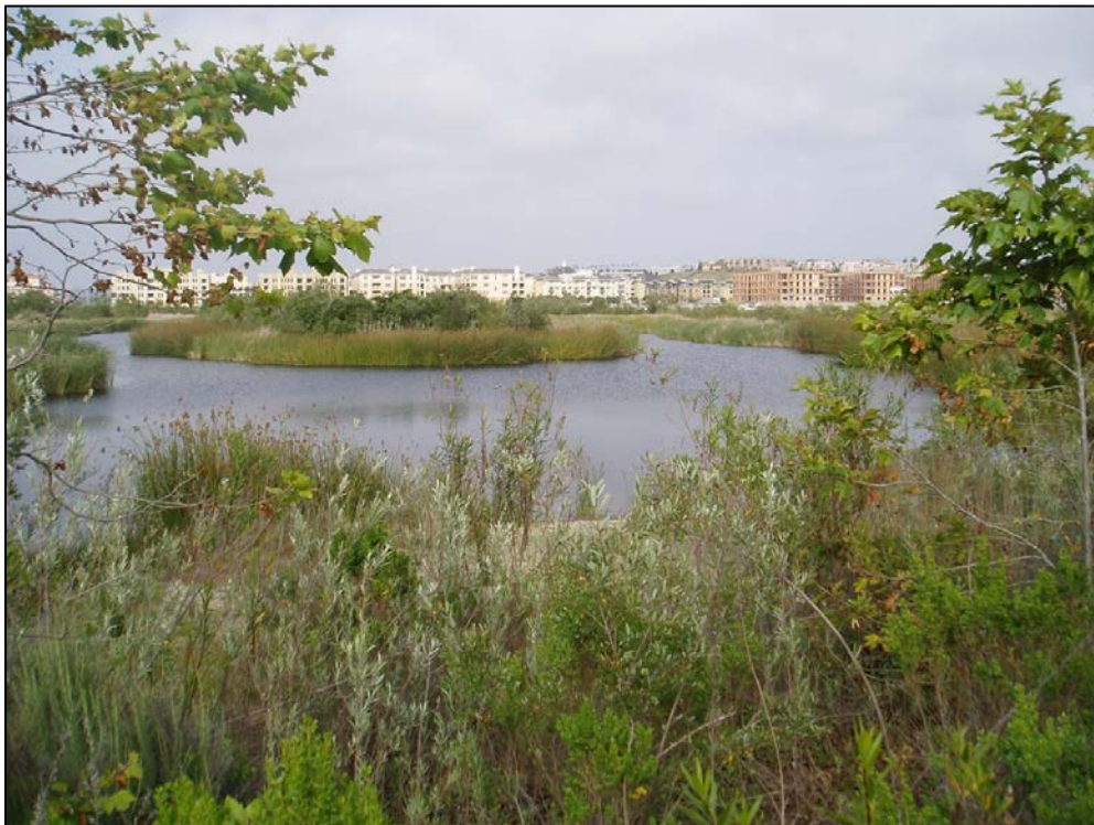
Figure 2: Example Constructed Southern California Wetland/Wet Pond (Photo: Geosyntec Consultants)
