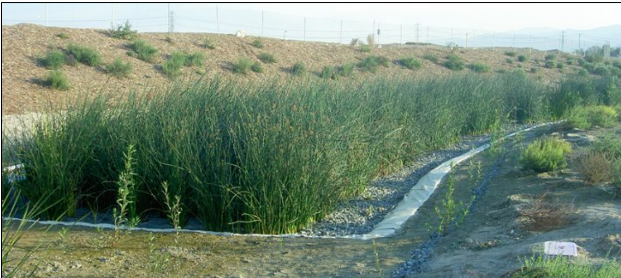
Figure 3: Example Subsurface Flow Wetlands (Photo: S. Lyon)
