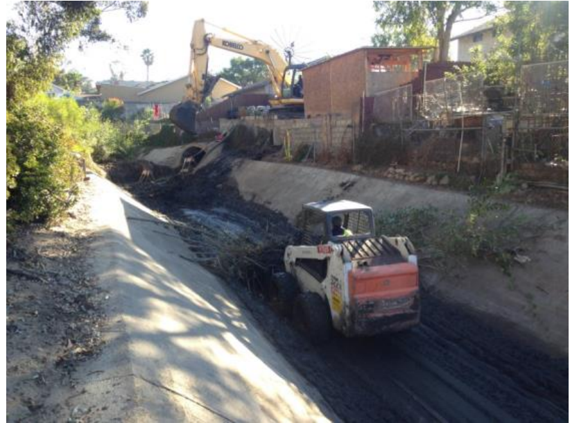
Photograph 6: Looking east from the north side of the channel at crew member using the bobcat to clear sediment and debris.
