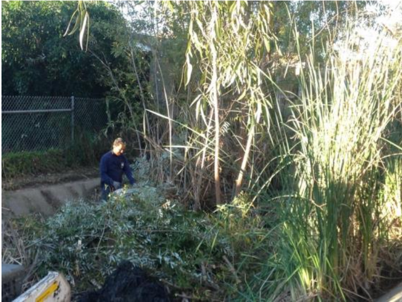
Photograph 5: Crew member using a chainsaw to clear large willows in the channel, channel is looking west.
