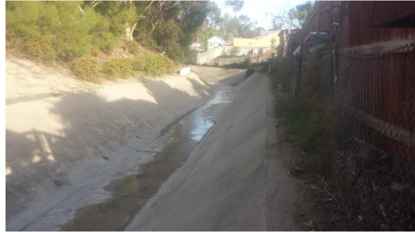
Photograph 10: Looking east from the south side of the channel following completion of maintenance activities.
