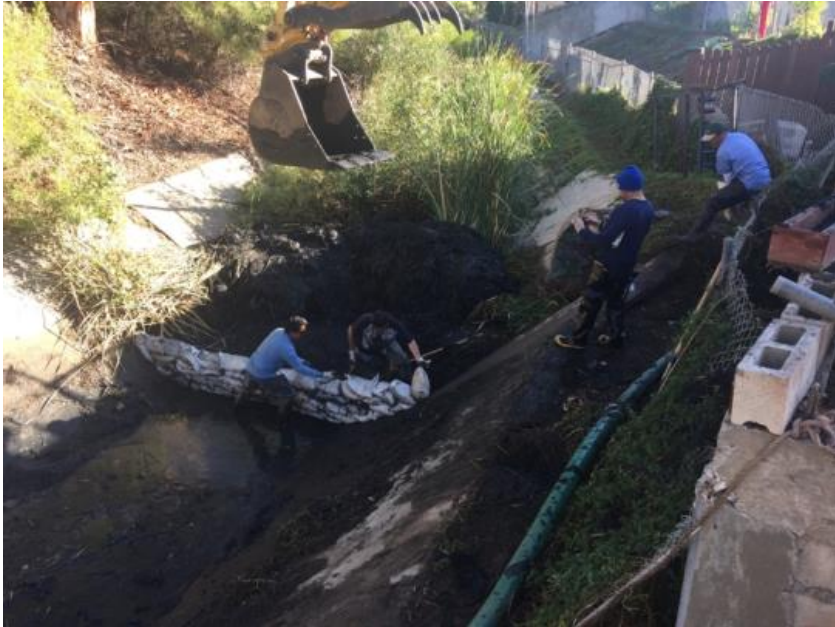
Photograph 3: Looking east into channel at crews building a sandbag berm within channel to keep water out of maintenance area to the west, channel is looking east.
