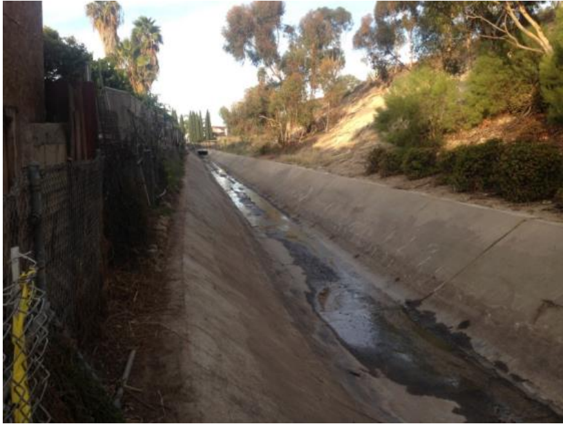
Photograph 9: Looking west from the south side of the channel following completion of maintenance activities.
