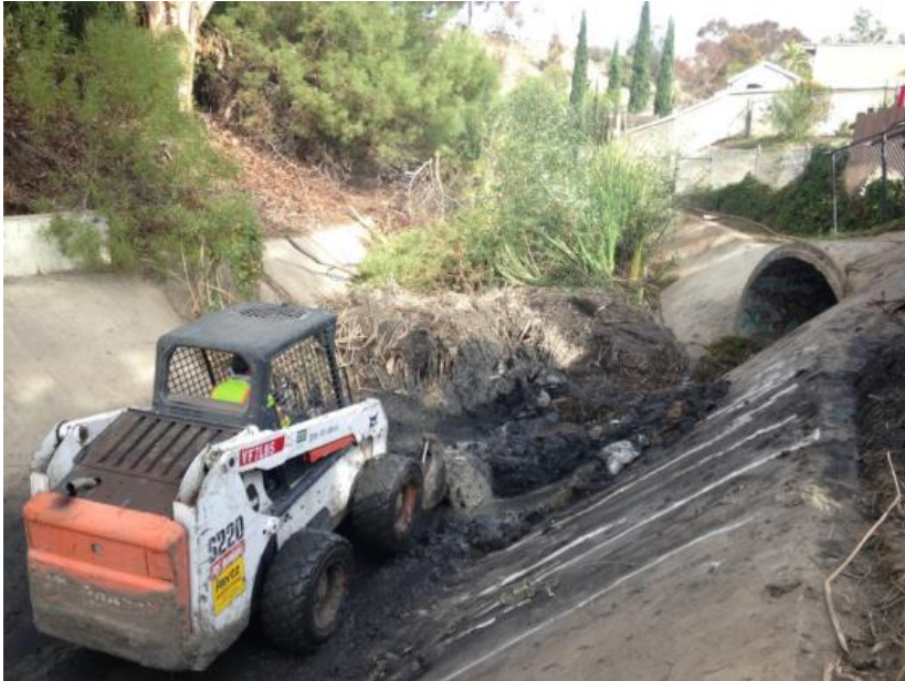
Photograph 7: Looking east from south side of channel at crew member using the bobcat to remove the sandbags from the water pumping area north of 4004 Via de la Bandola.
