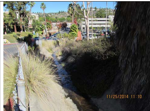
Photo 3: Downstream (facing north) looking toward inlet pipe, November 25, 2014.
