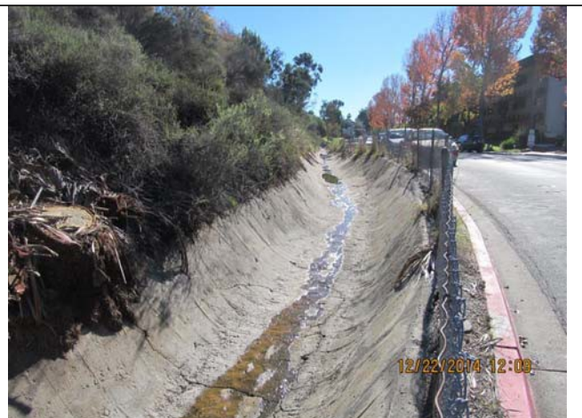
Photo 8: Upstream (facing south), December 22, 2014.
